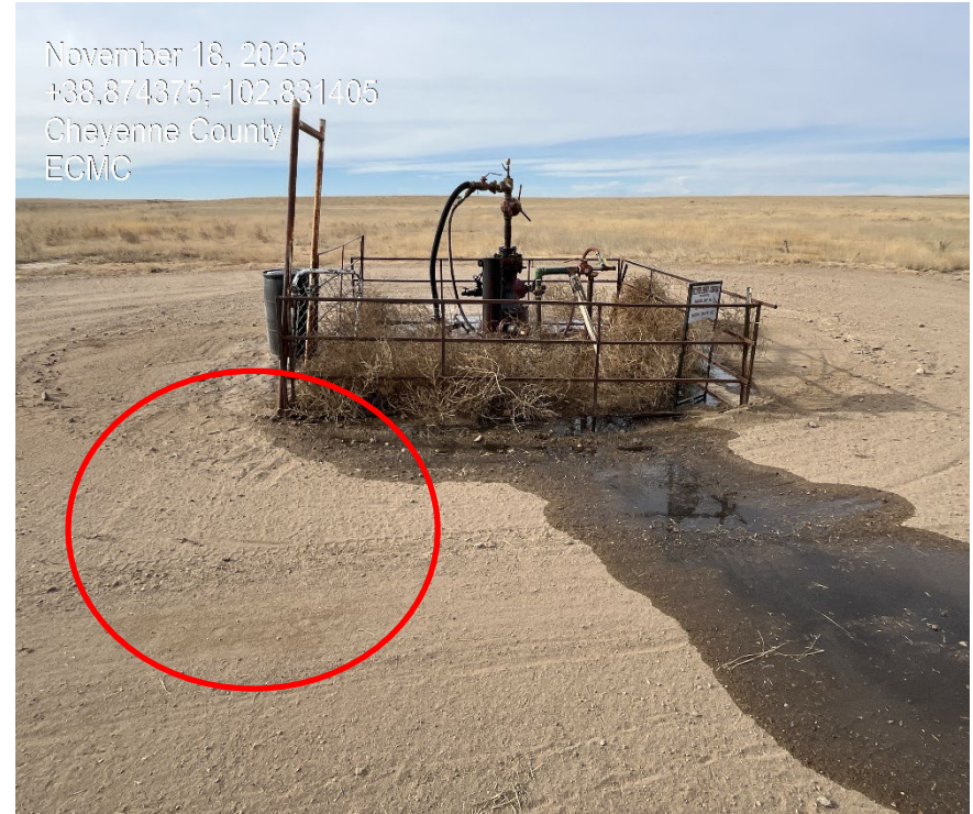
Photo 8. The next day when active sill was occurring, it was observed that the previous spill at area of red circle had been covered up with a drag harrow.
