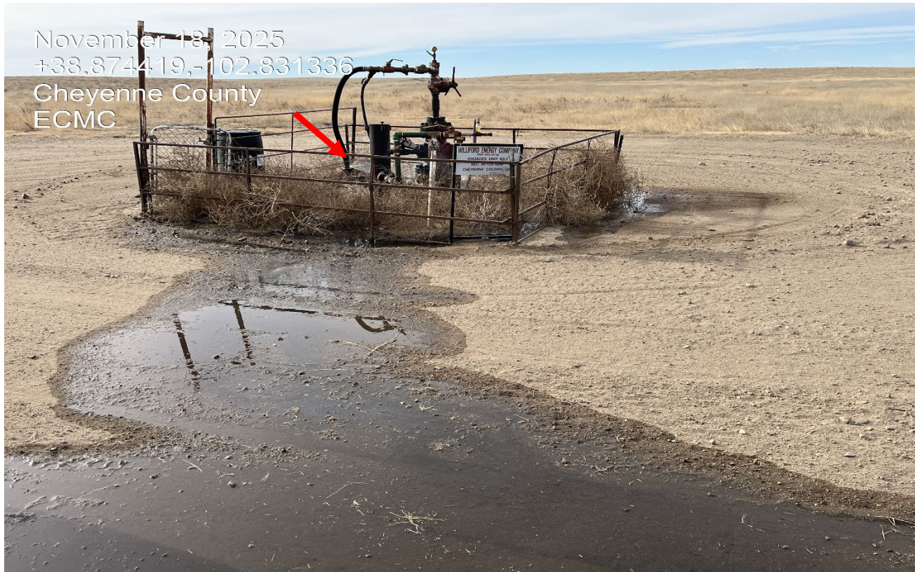
Photo 5. The source of the leak can be seen at red arrow..
