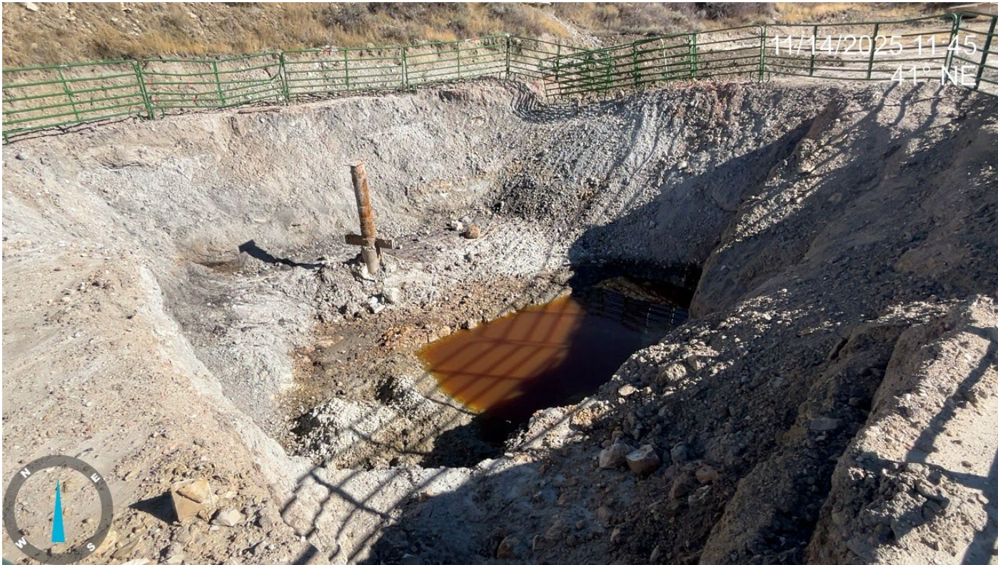
Photo 2: Photo showing the fenced and open excavation at the location.
