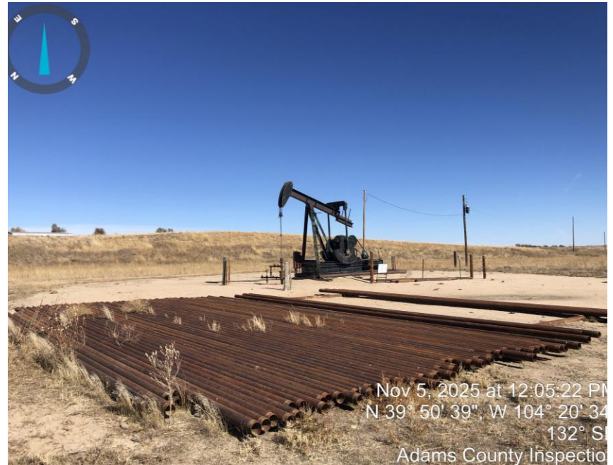
Photo #4 Pump jack & pipe.
