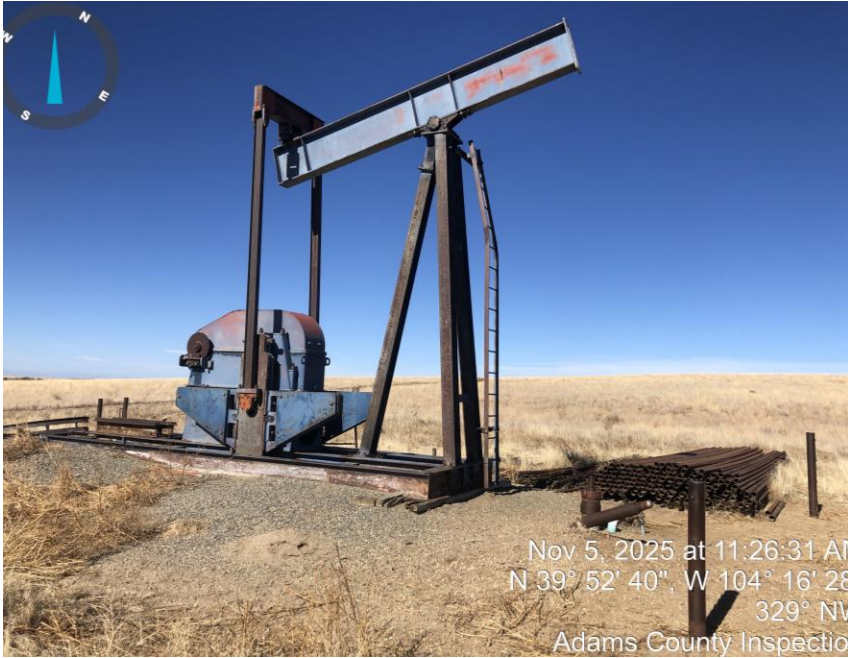
Photo #1 Pump jack & pipe.
