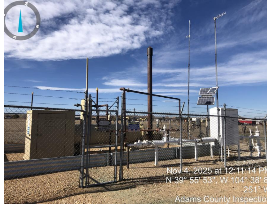
Photo #2 Separator & meter.
