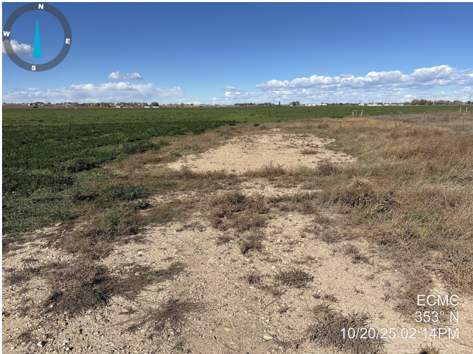
Photo 1. Photo taken of the tank battery location, facing north. Photo illustrates that location does not meet Rule 1004 standards as gravel, bare ground, and weedy annual vegetation were observed across the location.
