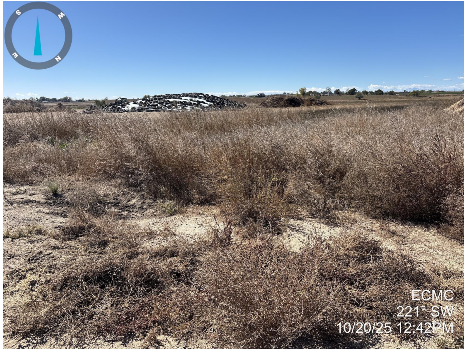
Photo 5. Photo taken of the tank battery location, facing southwest. Photo illustrates that the tank battery does not meet Rule 1004 standards as weedy annual vegetation was observed across the location.
