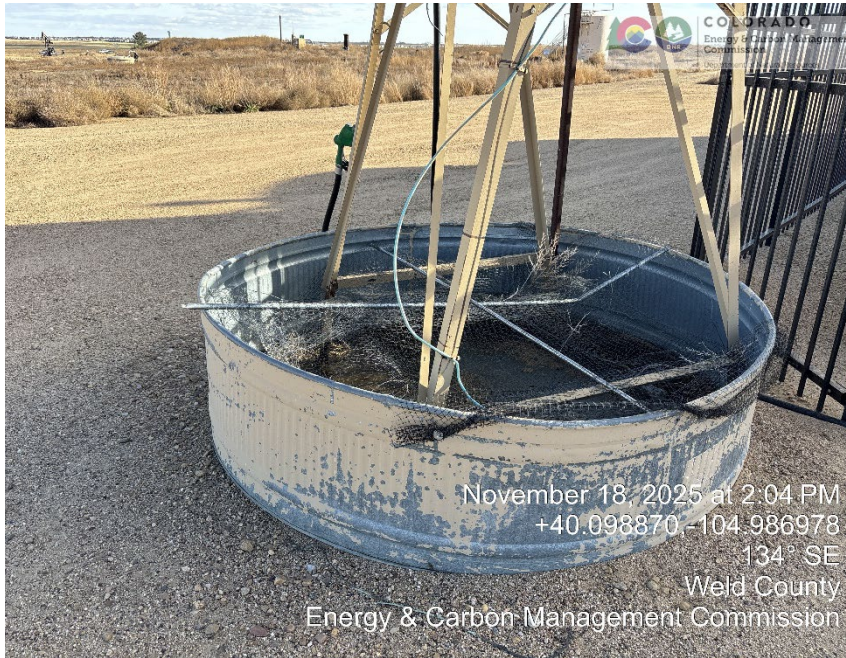
Methanol tank wildlife protection
