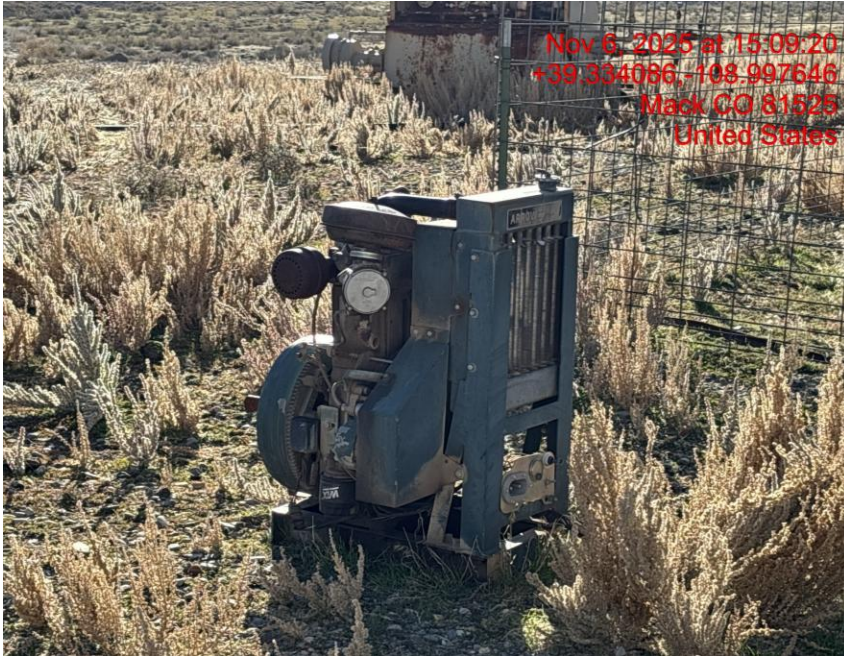
Stored/Unused Equipment/Weeds – Photo #01468
