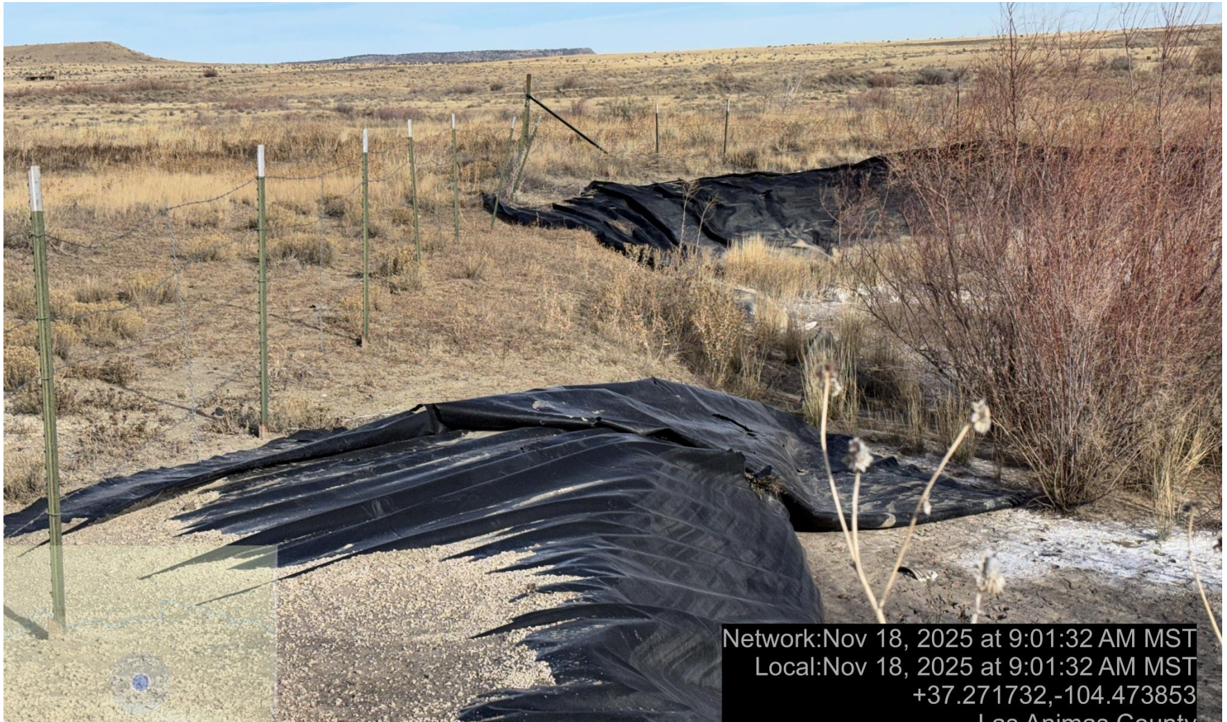
PHOTO 5: PIT LINER IS COMPROMIZED AND NOT MAINTAINED.
