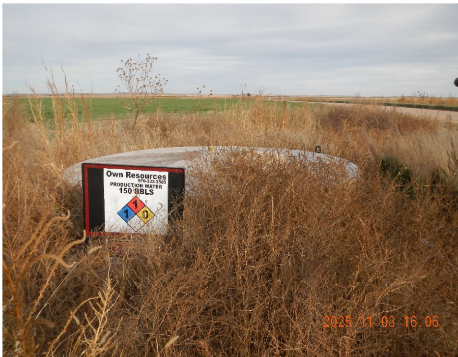
3. View of Production tank at remote gathering location. Note dried vegetation.
