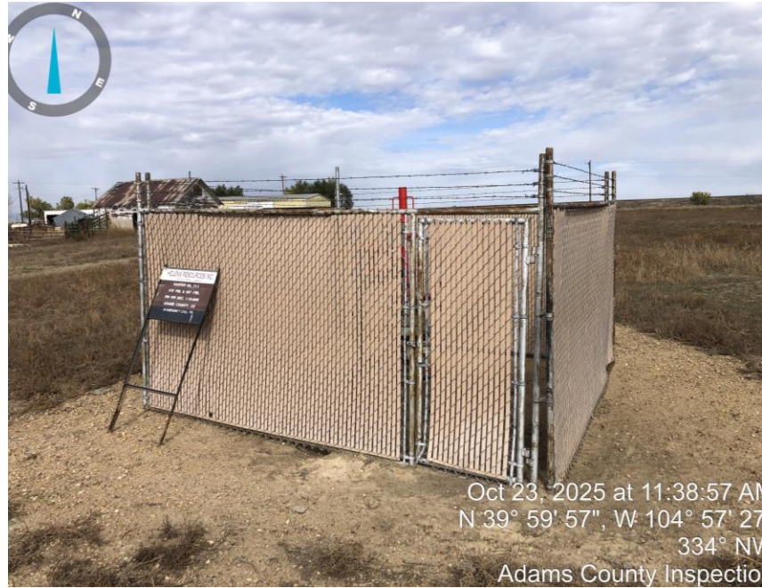
Photo #3 well head.
