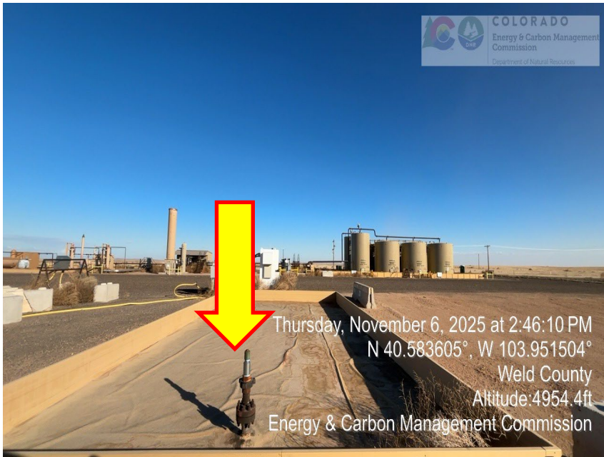
Photo 5 – Unmarked Riser
