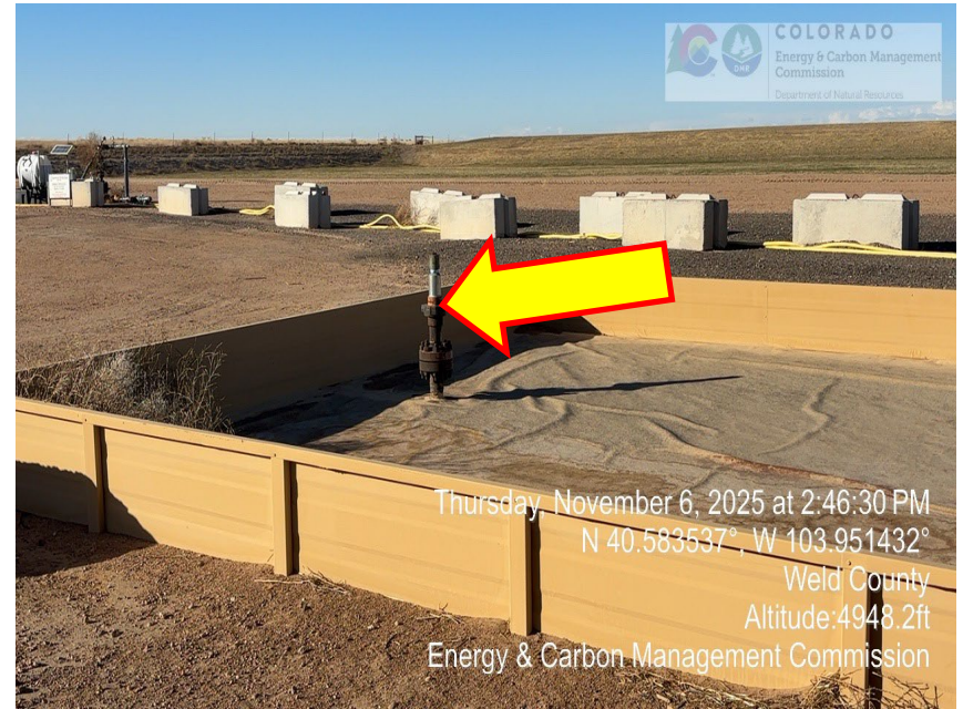
Photo 6 – Unmarked Riser
