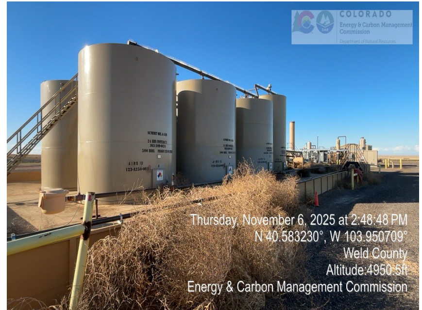
Photo 12 – Tank Battery
