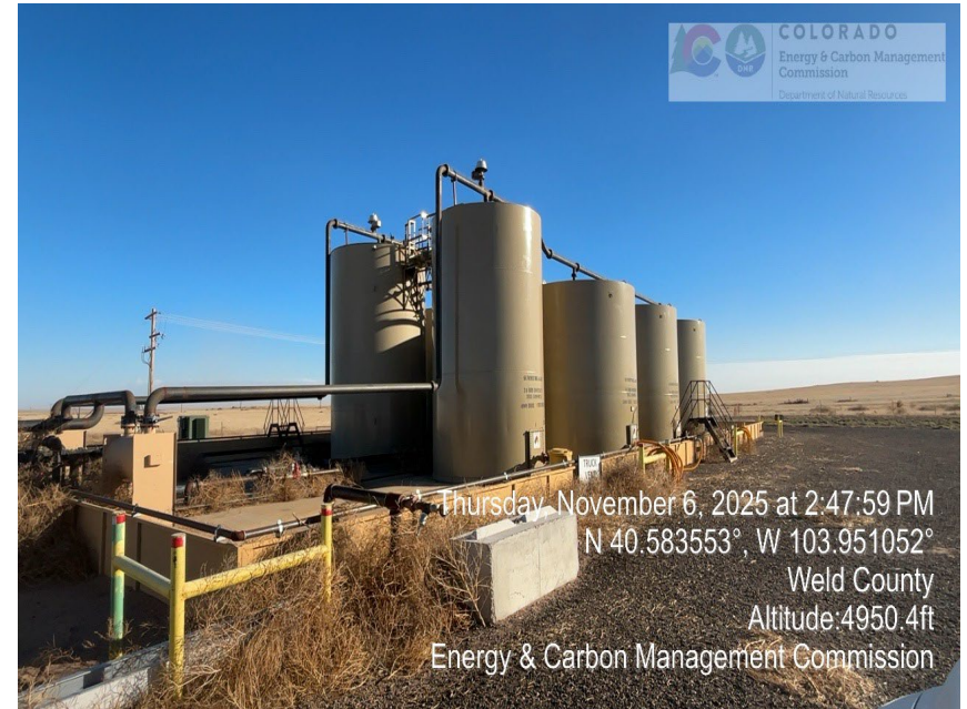
Photo 10 – Tank Battery
