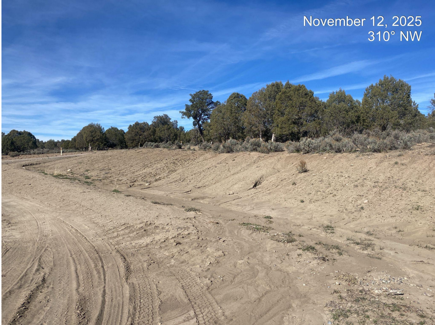
Photo 4. View of location northern cut slope which remains with bare loose soils and no vegetation establishment.
