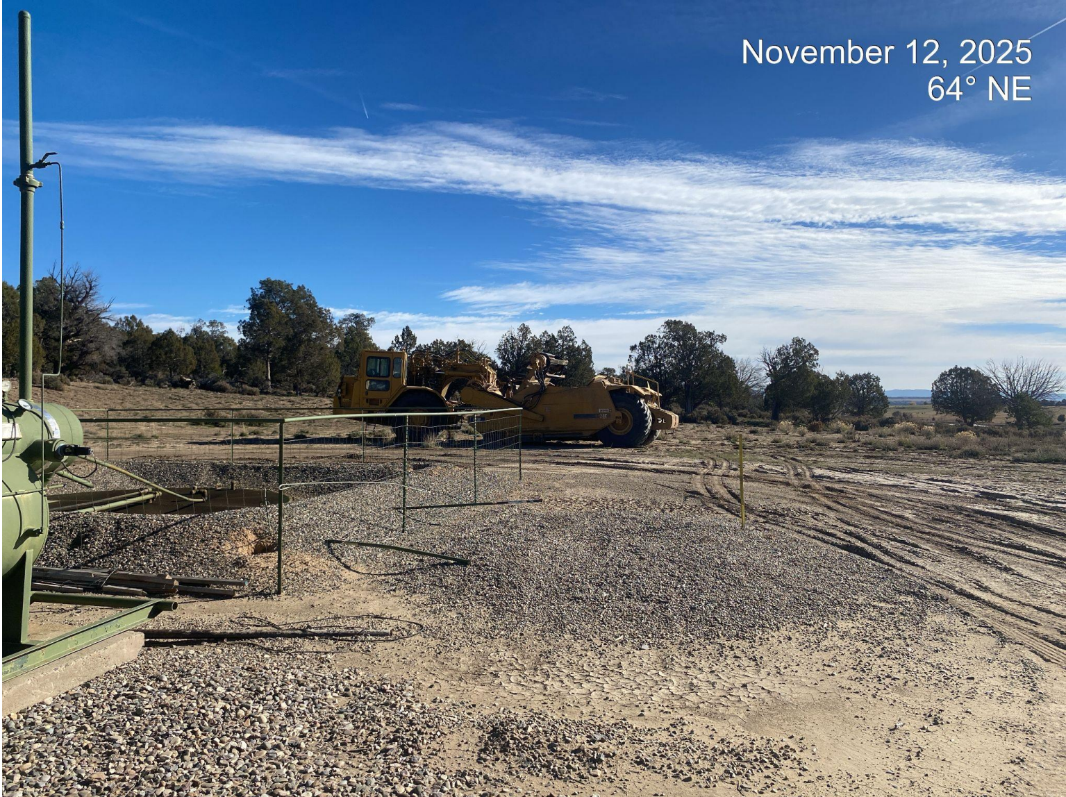
Photo 2. Unused shed on the location has been removed .
