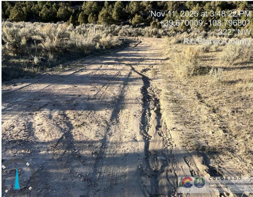
Photo # 4050 Insufficient erosion control on lease road; rill erosion cutting down lease road
