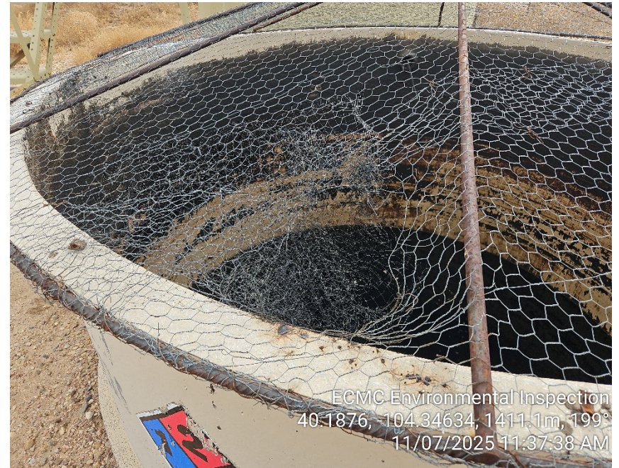
Photo 2 - Repairs to bird netting have torn on western produced water tank
