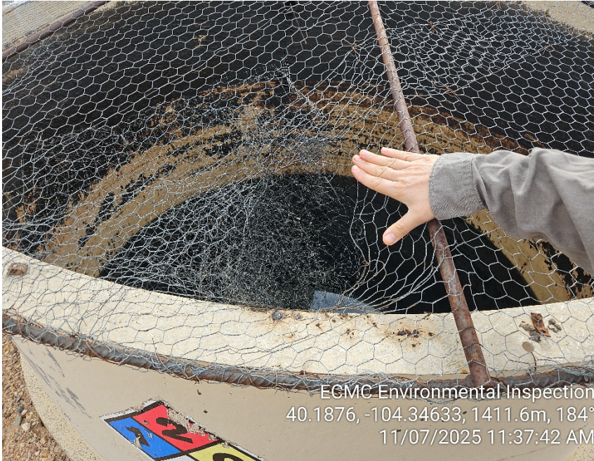
Photo 3 – Repairs to bird netting have torn on western produced water tank (hand for scale).
