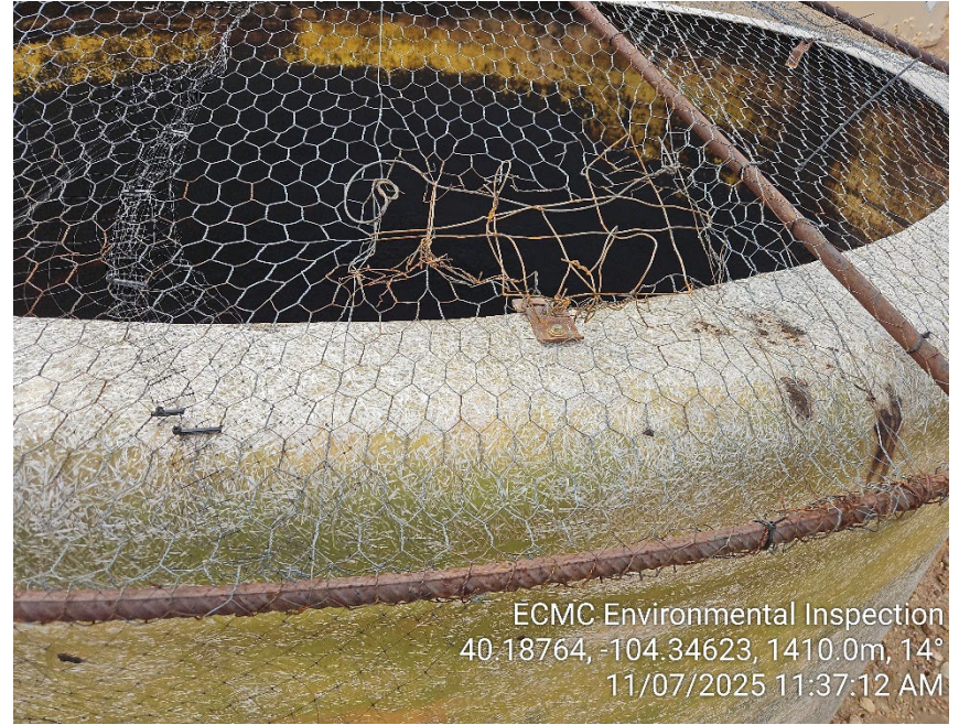
Photo 6 - Repairs on eastern produced water tank remain intact.
