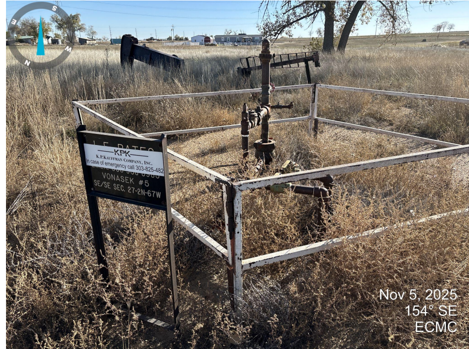
Photo 4. Photo taken at the wellhead. Undesirable weeds such as russian thistle present on location and touching equipment.
