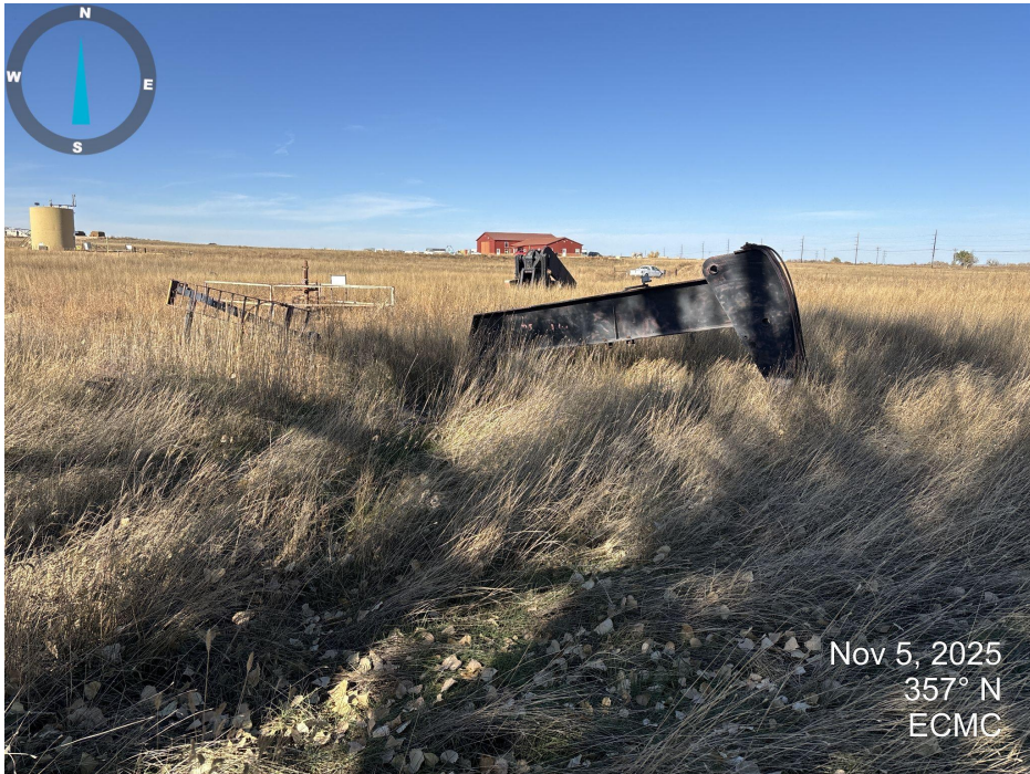
Photo 5. Looking north across the location. Disassembled pumpjack remains on location.
