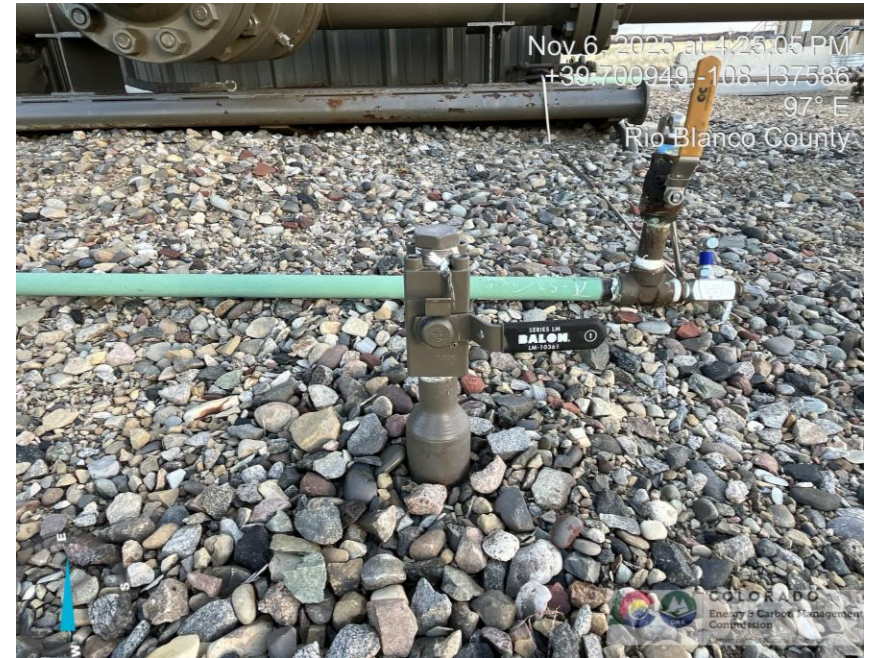
Photo # 3890 Unused flowline lacks lockout tagout (OOSLAT)
