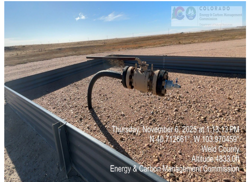
Photo 2 – Unmarked Riser
