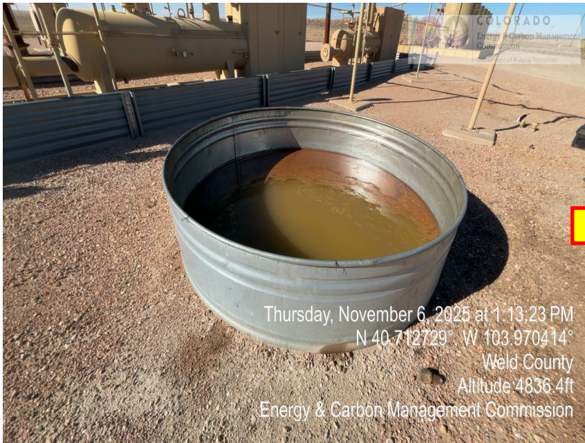
Photo 3 – Liquid inside unused Secondary Containment
