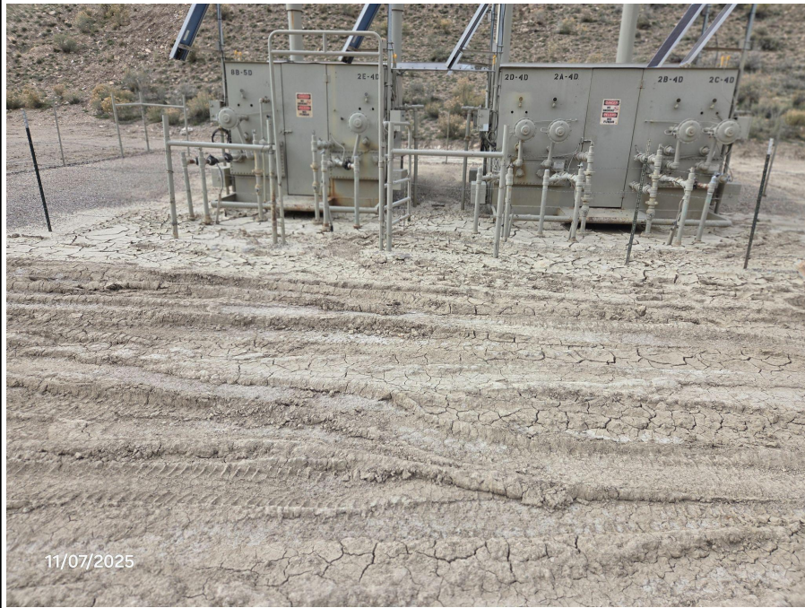
Photo 4: Photos taken from the separator equipment on the Location. See comments under photo 1. Photos also show evidence of ponding and comingling of stormwater with production equipment on the Location.
