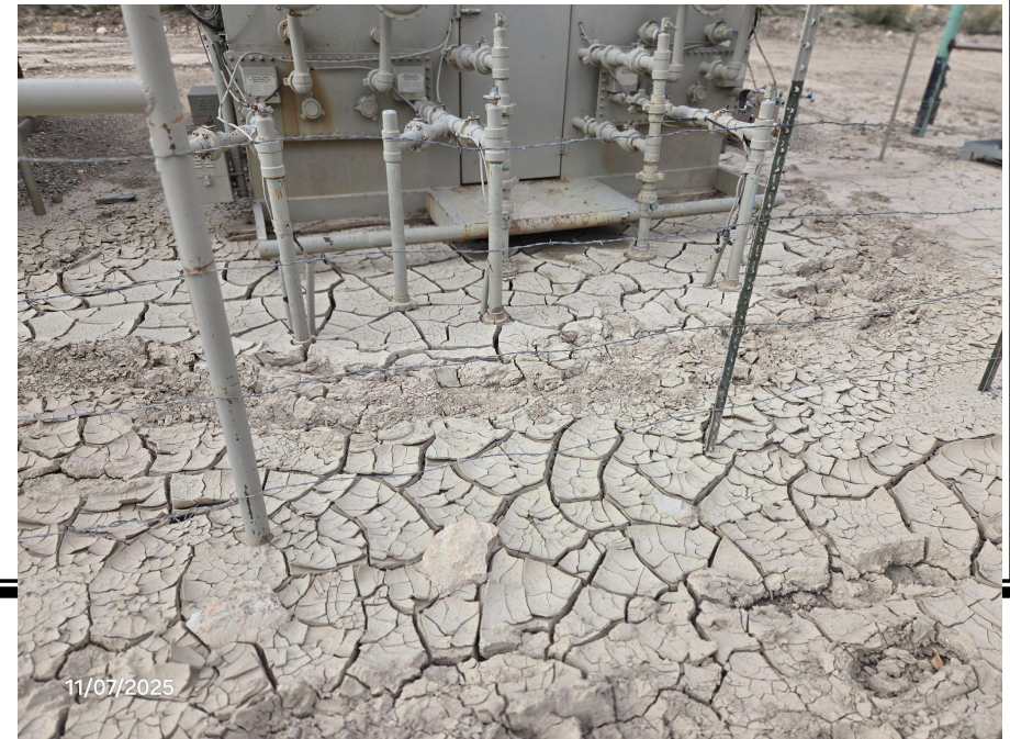
Photo 4: Photos taken from the separator equipment on the Location. See comments under photo 1. Photos also show evidence of ponding and comingling of stormwater with production equipment on the Location.
