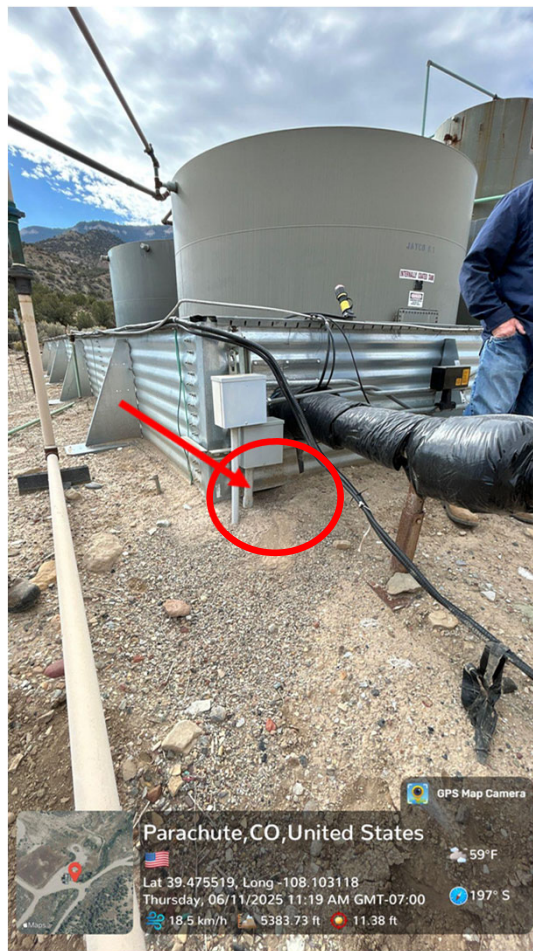
Photo 8 – Wildlife burrow under containment
