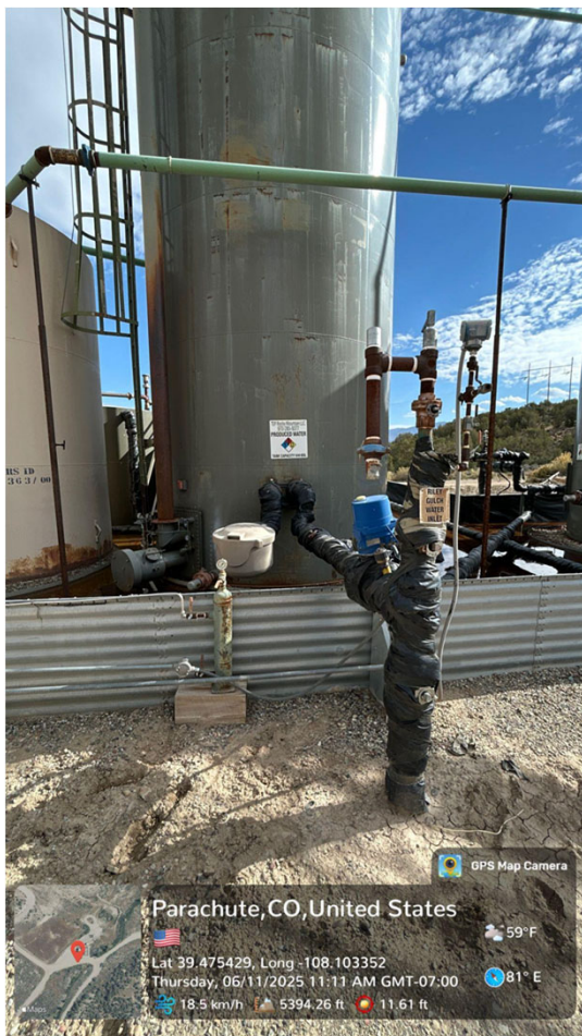
Photo 7 – Facing East from West Side of Tank Battery
