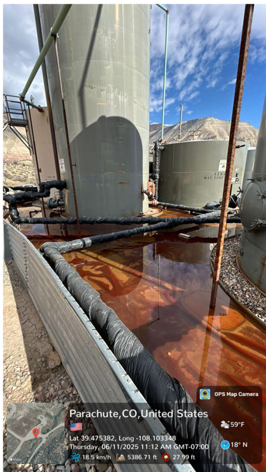
Photo 4 – Standing water in containment area at Tank Battery
