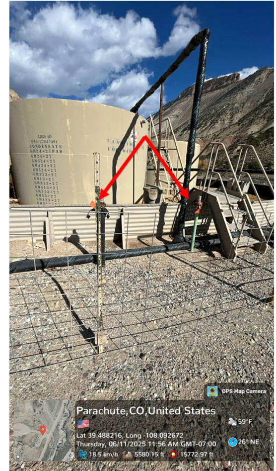
Photo 6 – Facing Northeast of Tank Battery
