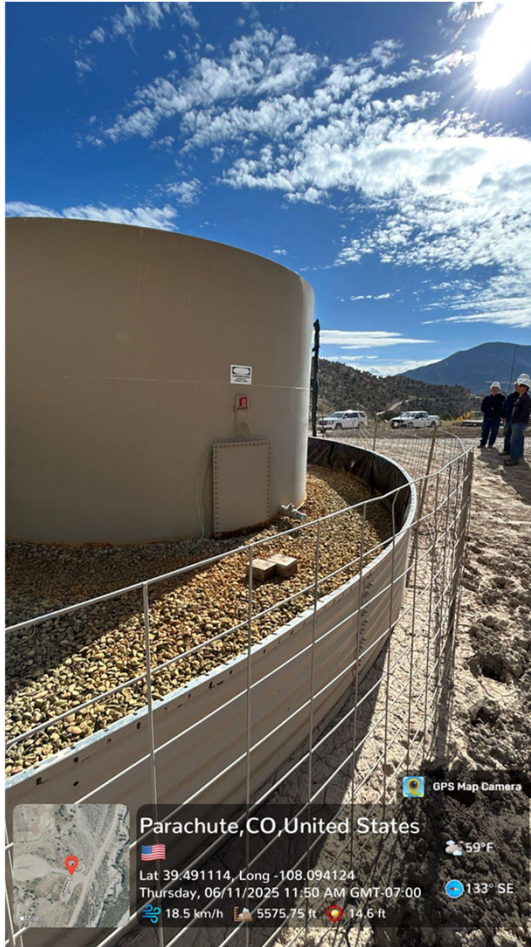
Photo 4 – Facing Southeast view of hydrovaced spill area
