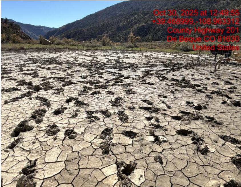
Lack of Stabilization – Photo #01325
