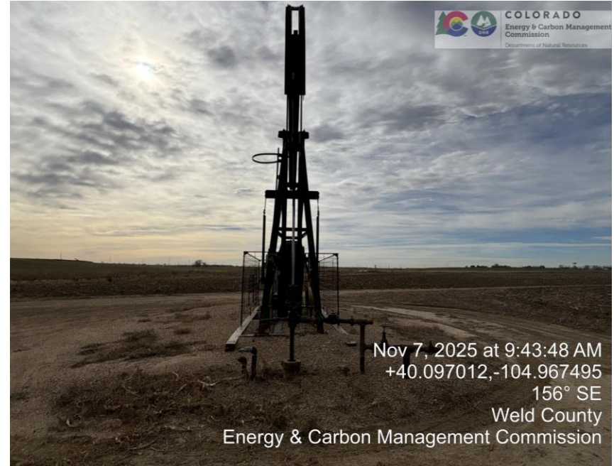
Photo 2 well head and equipment
