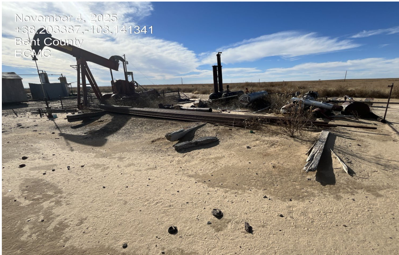
Photo 10. Facing southwest at the wellsite. There are various unused equipment, pipe, and debris stored on location that needs to be removed.
