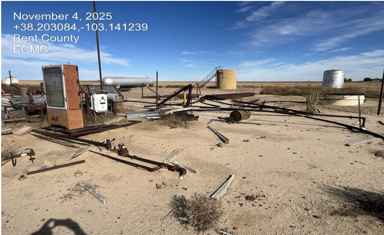
Photo 15. Facing northeast the location with various unused equipment, supplies and debris laying on the ground.
