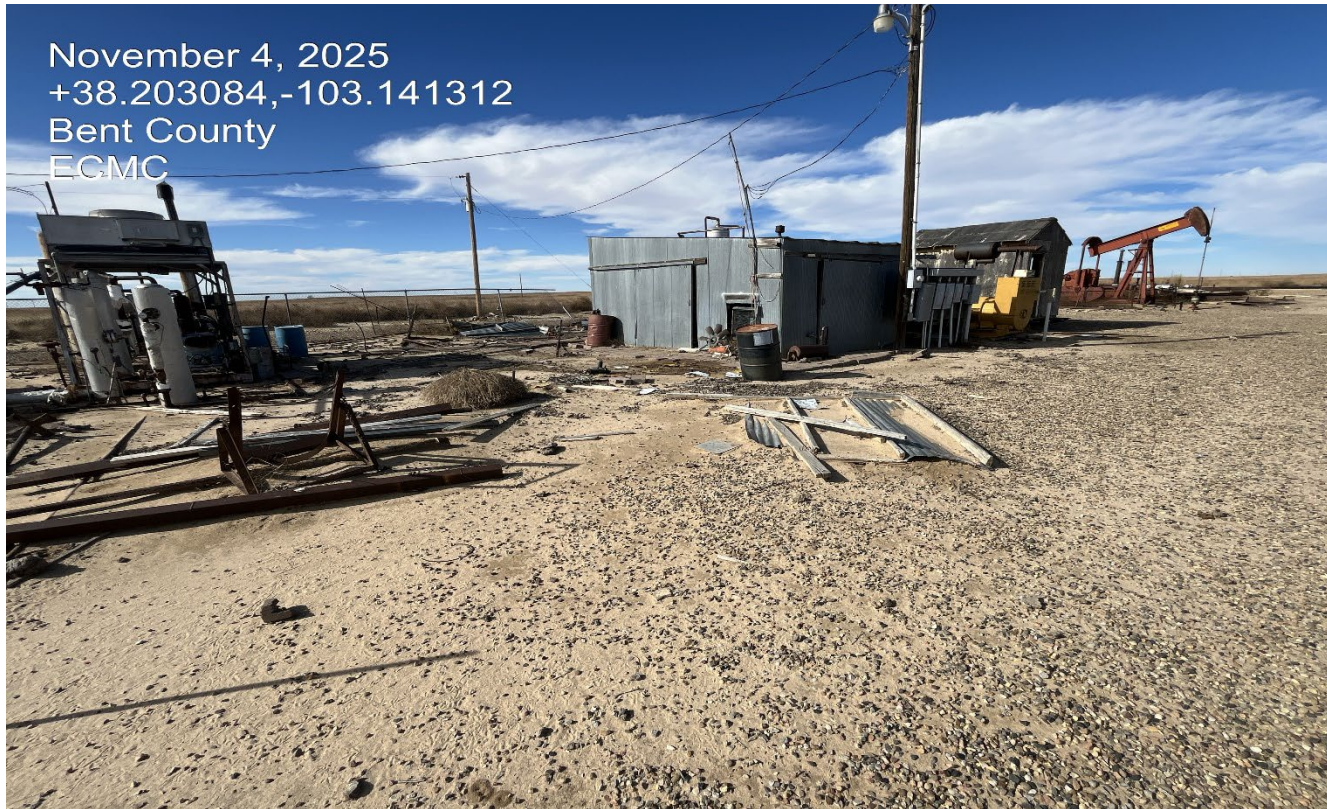
Photo 3. Facing northwest toward the GAS PROCESSING PLANT and Wellsite. There is various supplies and debris scattered throughout the location.
