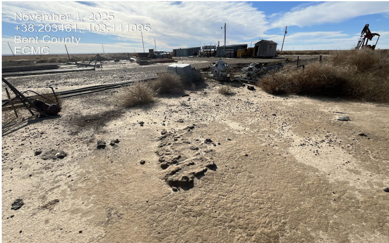
Photo 12. Facing southwest at the location. There is various unused equipment, supplies and tanks stored at the location that will need to be removed. The soils in this area are stained with hydrocarbon impacts from historic spill.
