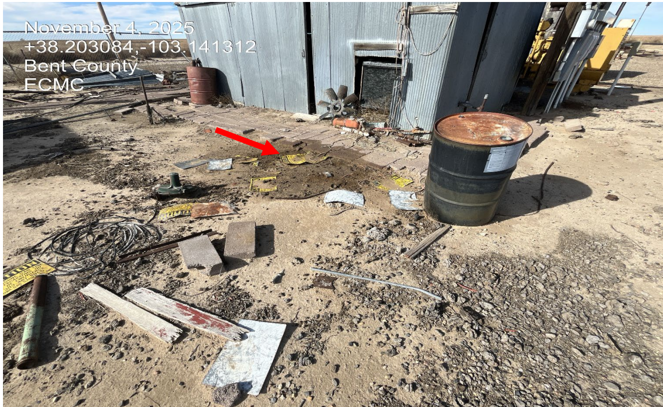
Photo 4. Facing northwest at the sheds and various equipment which are in disrepair. There is still oil stained soils from the barrel that leaked out shown at red arrow.
