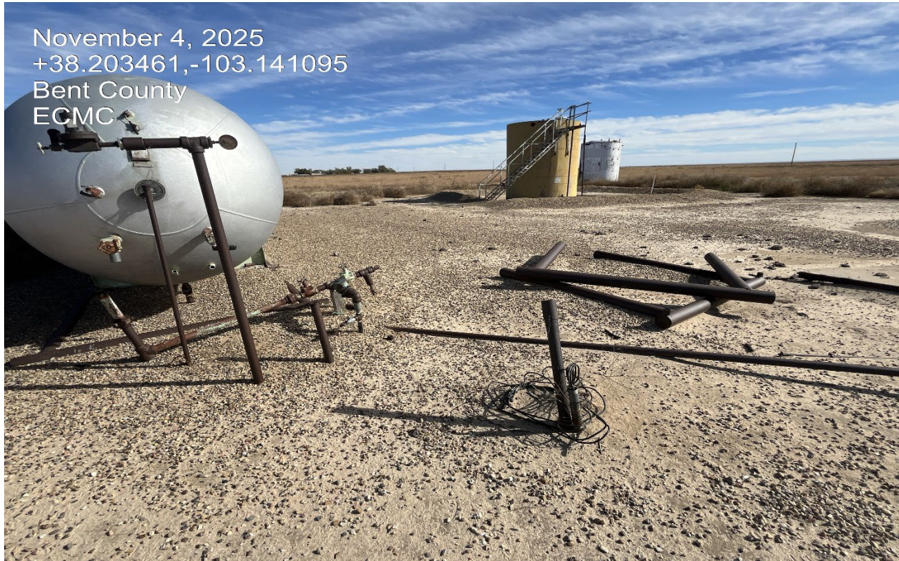
Photo 13. Facing southeast at the location. There is various unused equipment, supplies and tanks stored at the location that will need to be removed.
