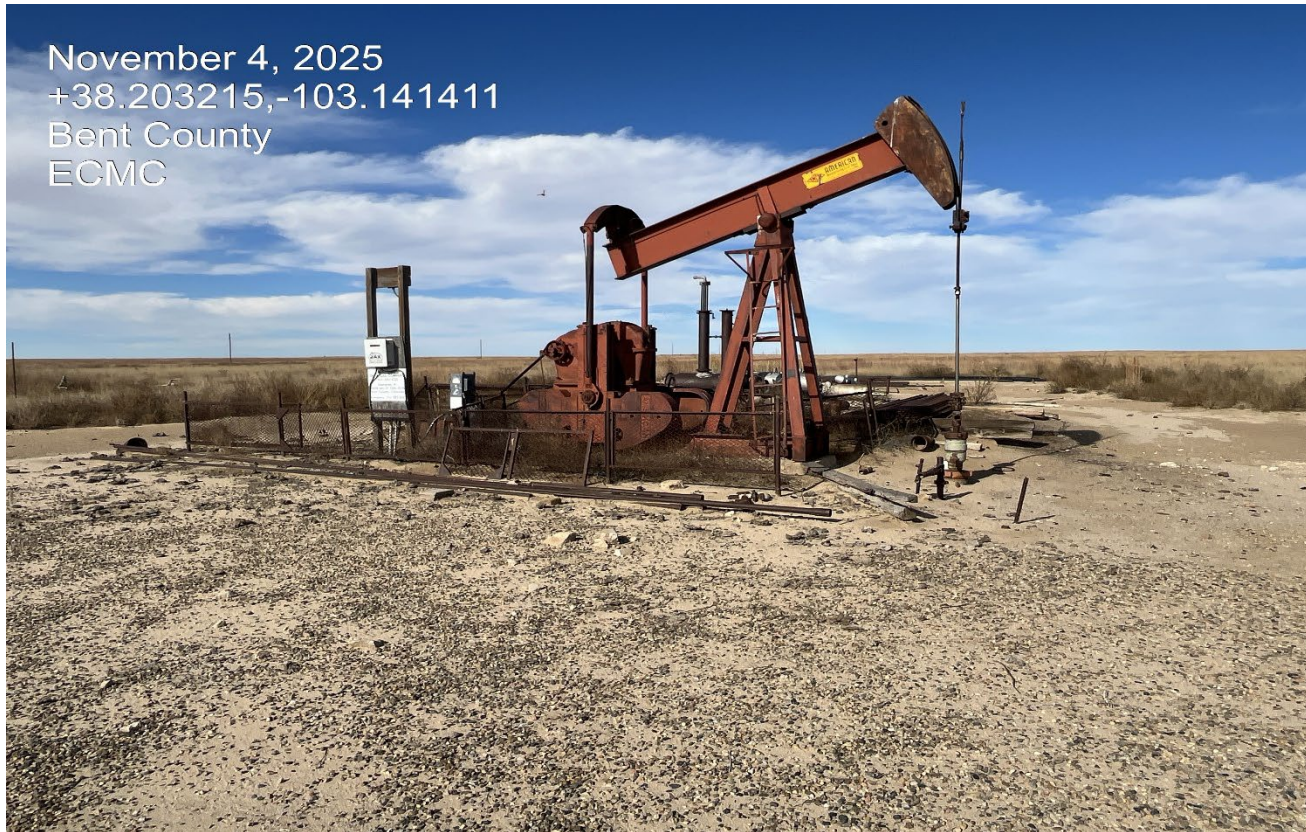
Photo 9. Facing northeast toward the well. The fence around the pumpjack is in disrepair and there is unused equipment stored near the well.
