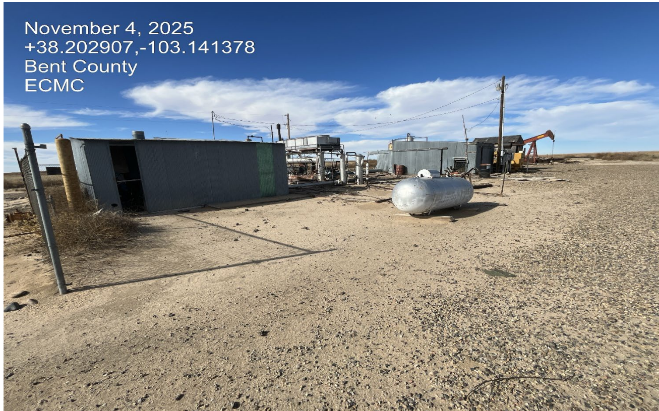
Photo 2. Facing northwest toward the GAS PROCESSING PLANT and Wellsite.
