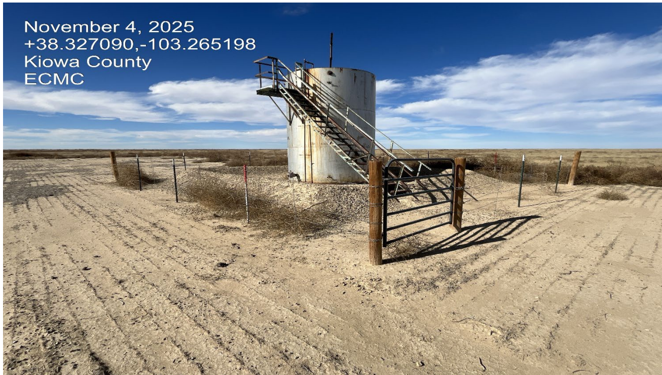
Photo 4. Facing toward the tank which is fenced and maintained. Currently not in use since well is TA'd.
