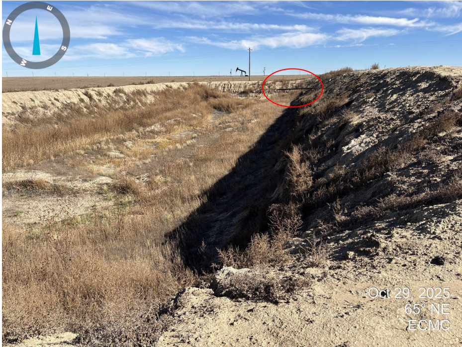
Photo 7. Looking east across pit #117577. Overflow pipe remains (red circle).
