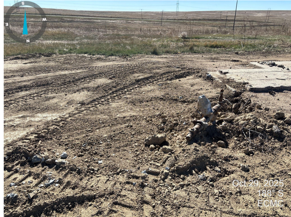
Photo 10. Excavation around the wellhead is filled in. A pipe riser remains.
