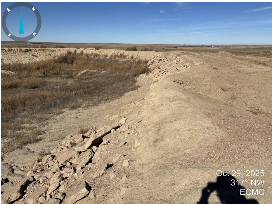
Photo 3. Looking northwest across the storage tank area along the east side of the pit. Concrete rubble is present.
