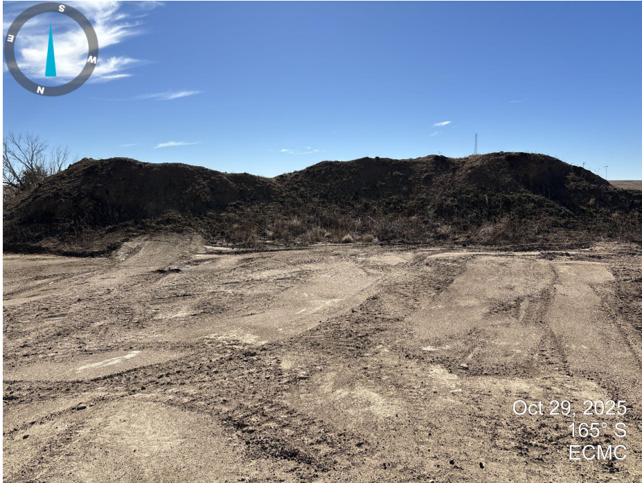
Photo 5. Soil pile near pit ID 440212 does not have stormwater protection BMPs.
