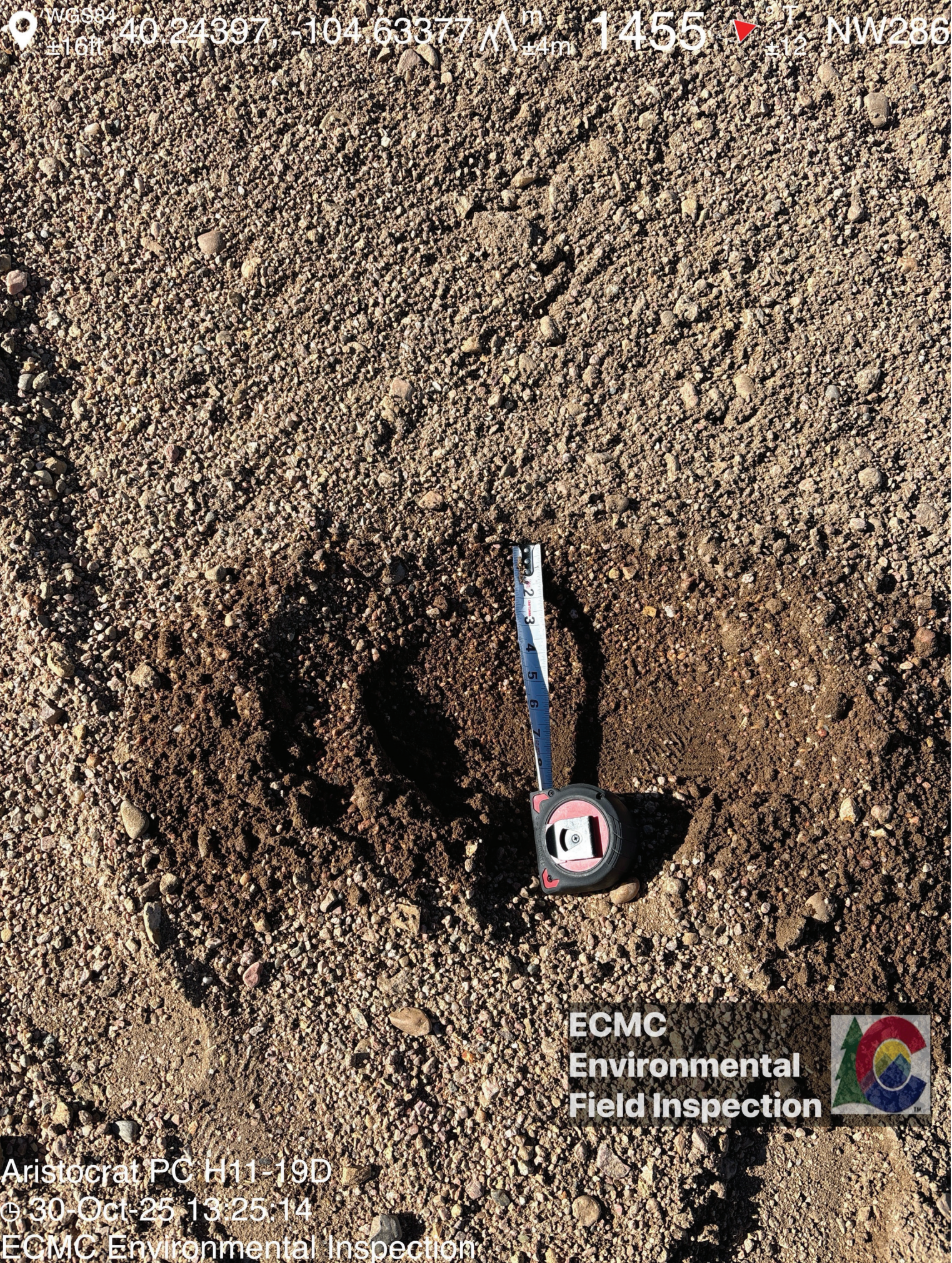
Pea gravel and soil used as backfill.
