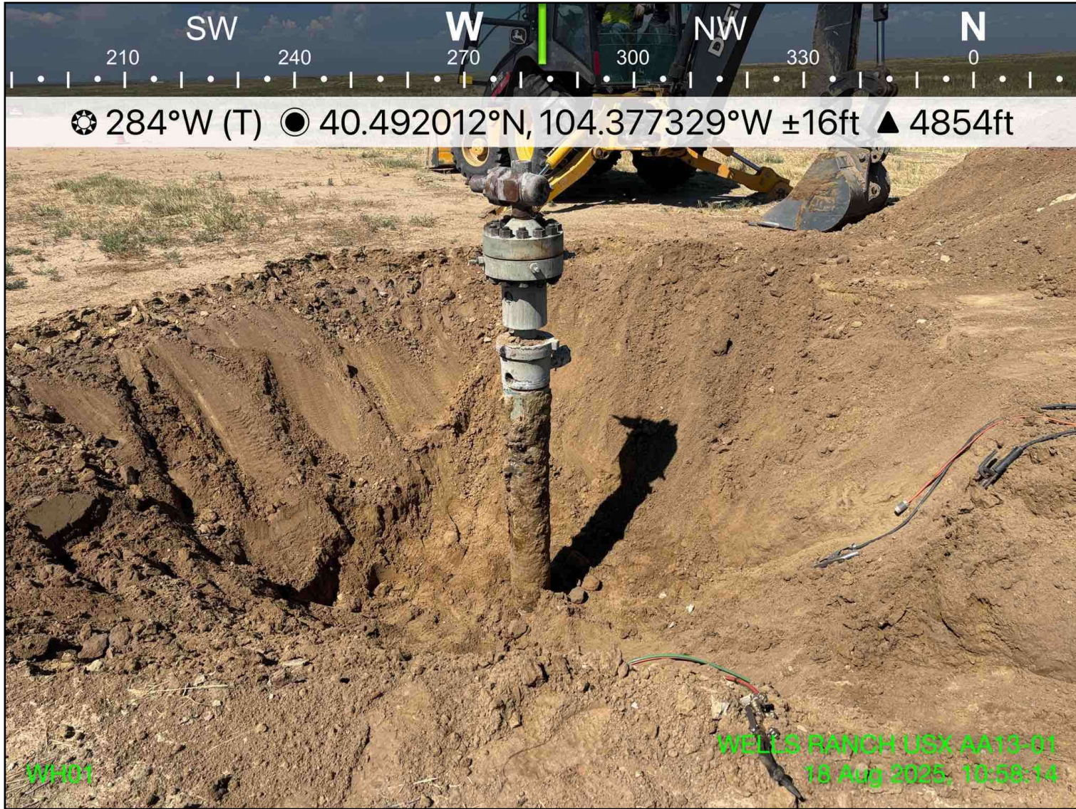
Photo 1: View of WH01 sample location and excavation extent, facing west
