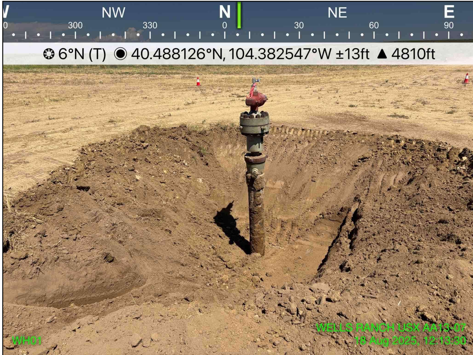
Photo 4: View of excavation extent, facing north
