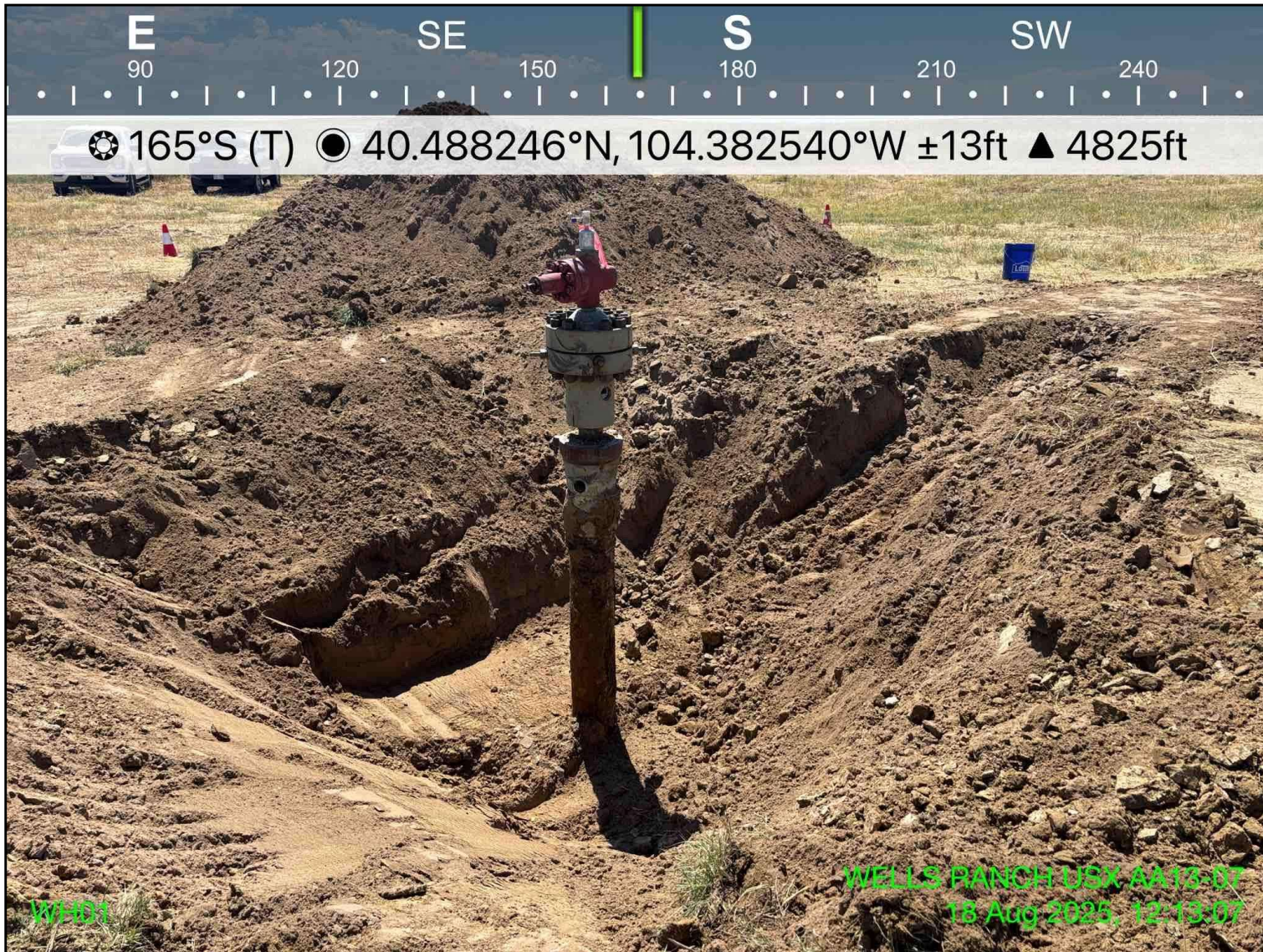
Photo 2: View of excavation extent, facing south
