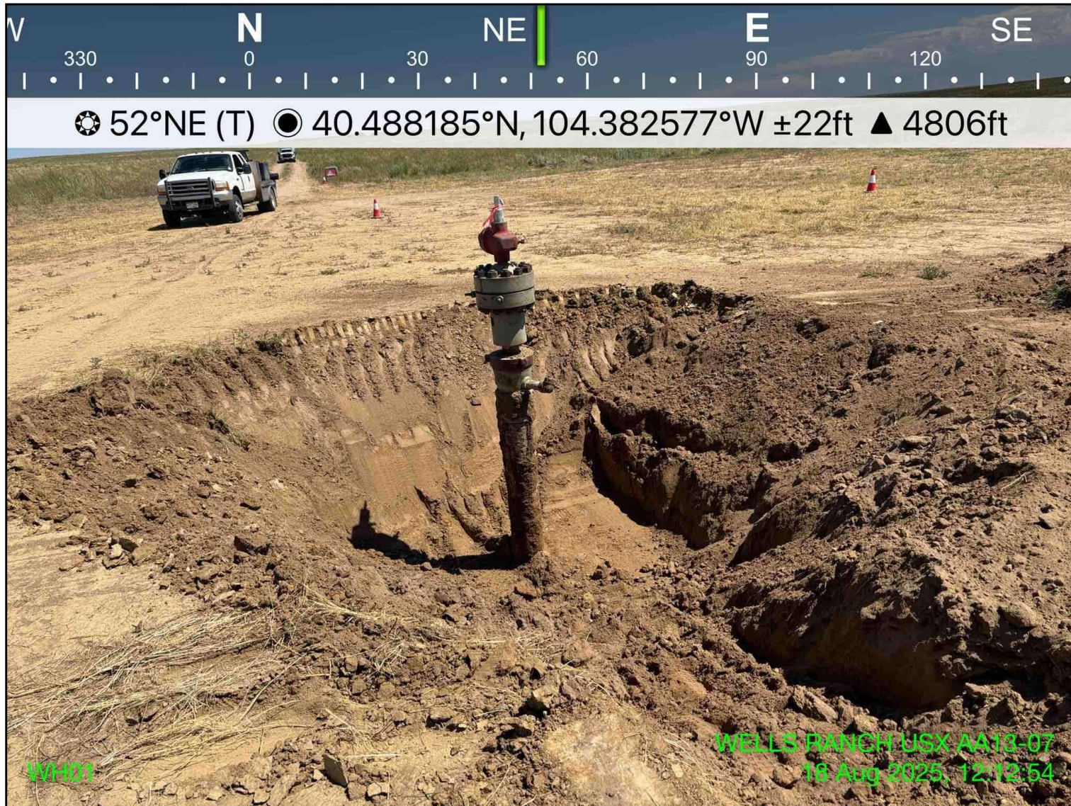
Photo 1: View of excavation extent, facing northeast
