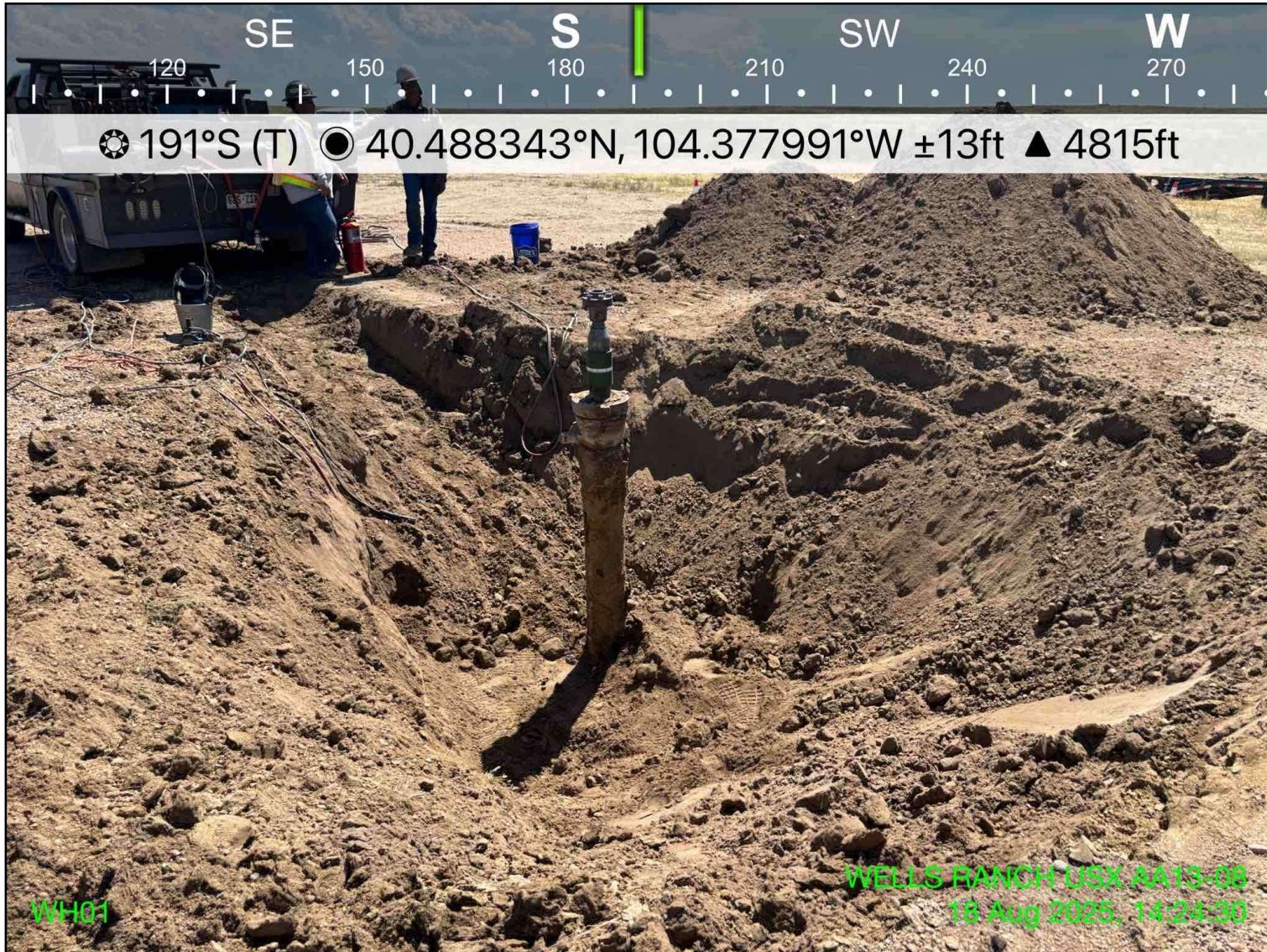
Photo 3: View of WH01 sample location and excavation extent, facing south
