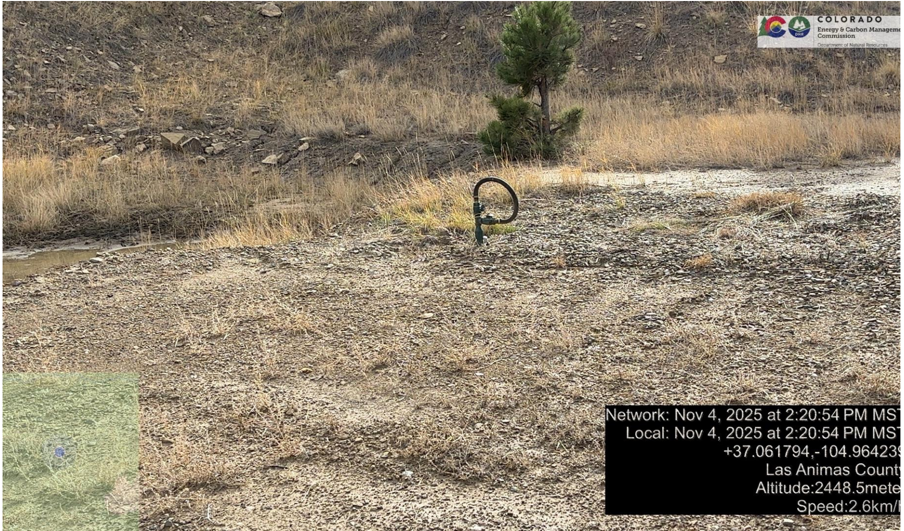
PHOTO 5: UNUSED EQUIPMENT ( 1" RISER NEAR WELLHEAD).
