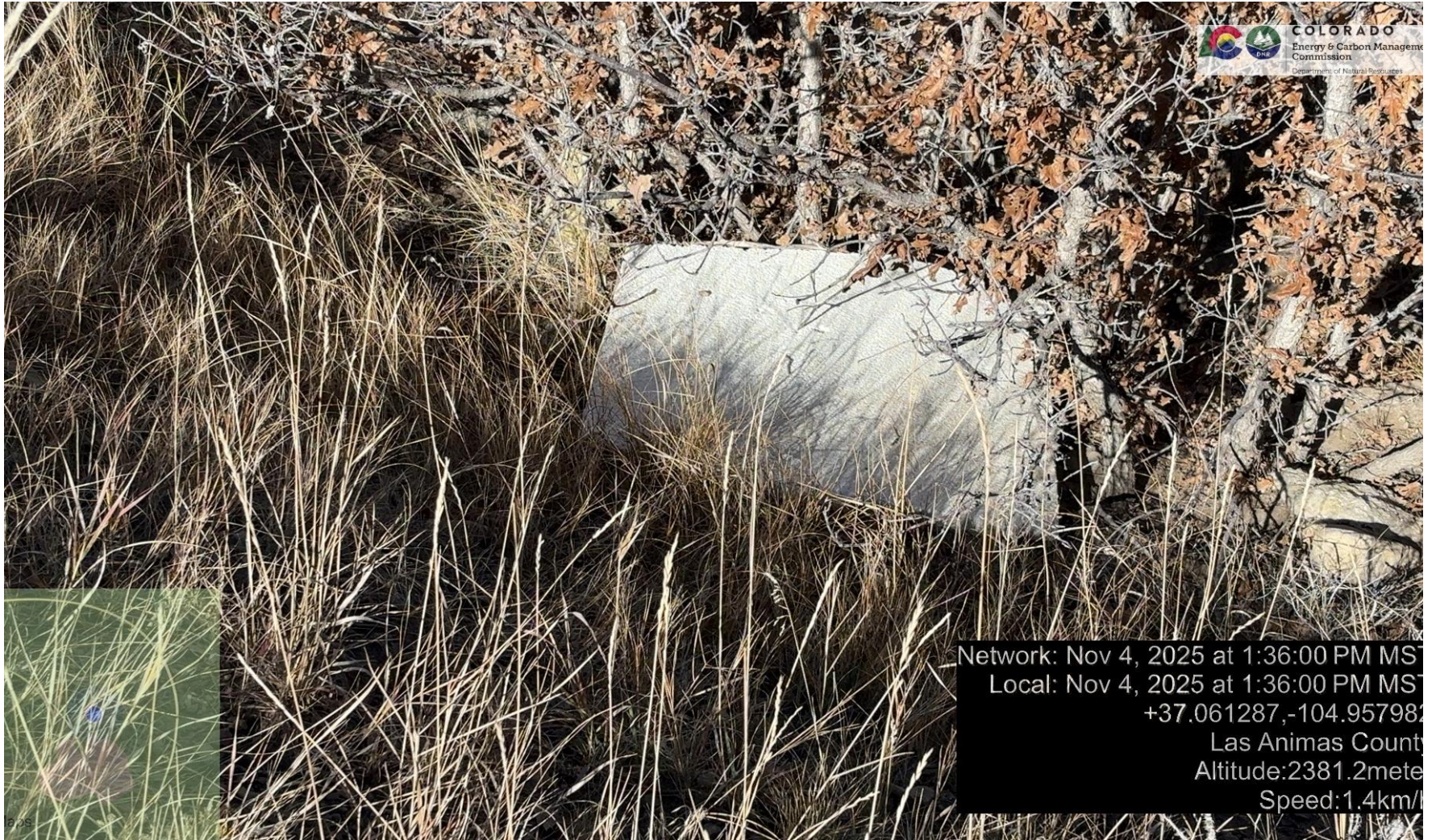
PHOTO 3: TRASH OFF THE NORTH END OF LOCATION. REMOVE ALL TRASH FROM LOCATION PER RULE 606. CA DATE 11-14-2025.
