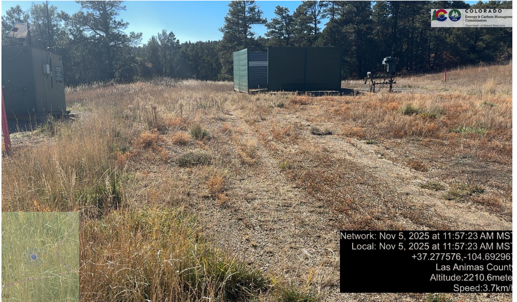
PHOTO 3: WEEDS NOT MAINTAINED. MAINTAIN WEEDS PER RULE 606. CA DATE 11-15-2025.
