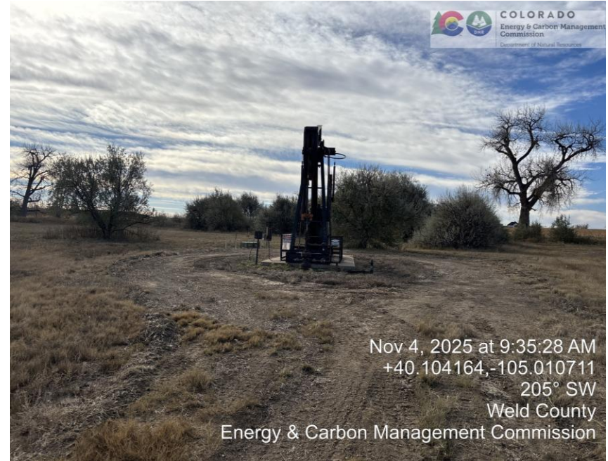
Photo 2 well head and equipment
