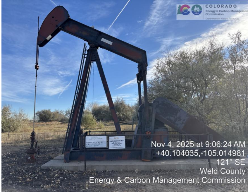
Photo 1 well head and equipment
