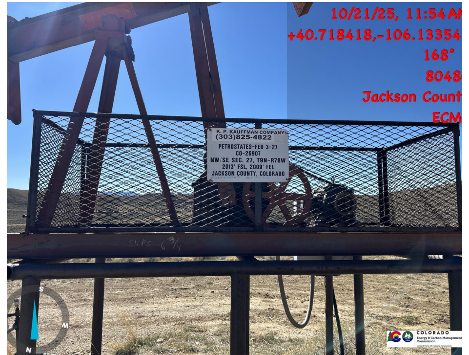
Well signage lacks information
