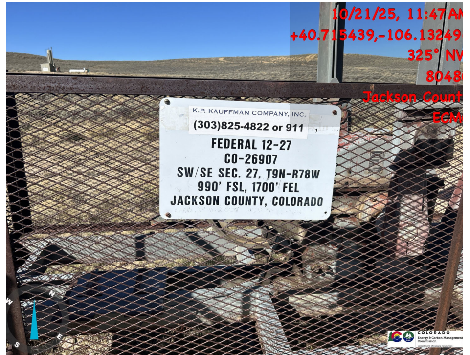
Well sign lacks information
