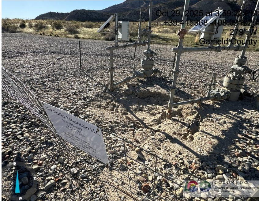
Photo # 4118 Subsidence developing near Williams SG 531-27 wellhead
