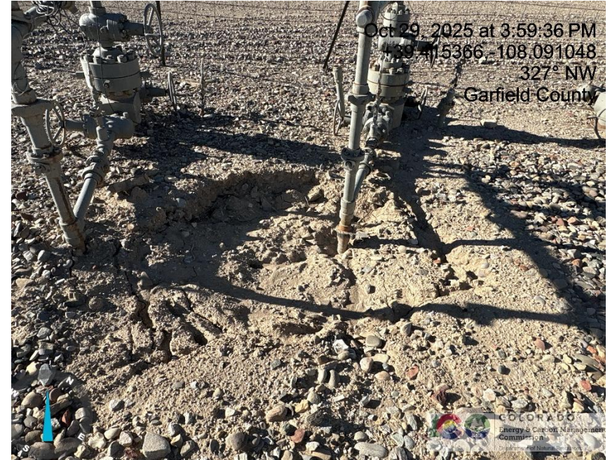
Photo # 4119 Subsidence developing near Williams SG 531-27 wellhead
