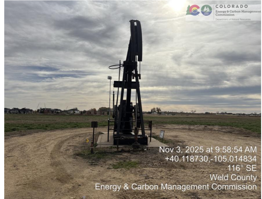
Photo 2 well head and equipment
