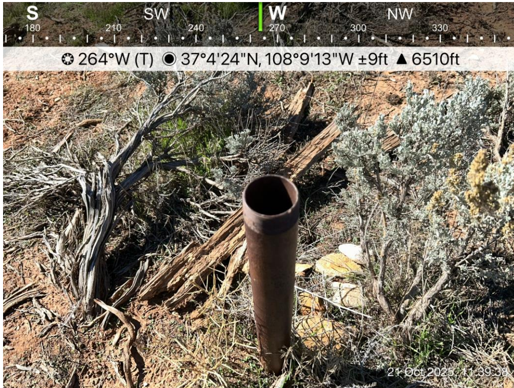
Photo 2: Taylor #3-B (OWP) Wellhead.
