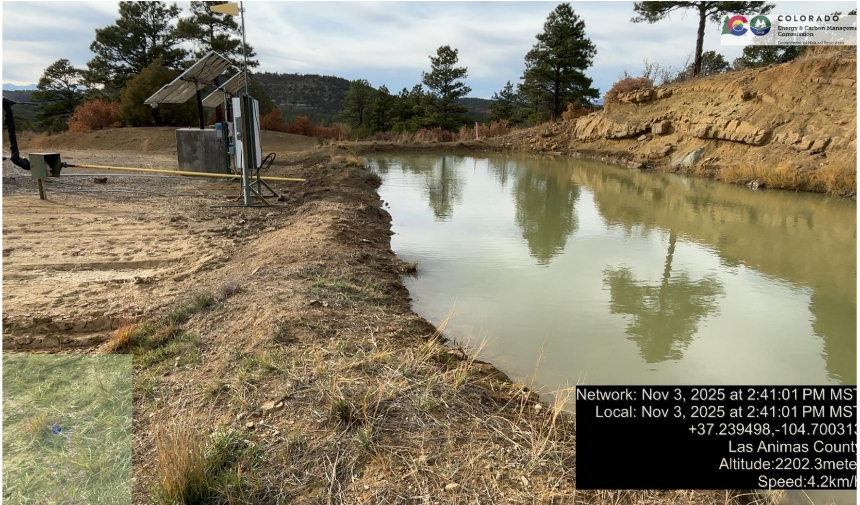
PHOTO 3: Less than 2-feet of freeboard (FREEBOARD IS MEASURED FROM ORIGINAL GROUND LEVEL NOT TOP OF BERMS). LEFT A PHONE MESSAGE WITH OPERATOR. Lower fluid level so at least two feet of freeboard exists per Rule 909.c.
