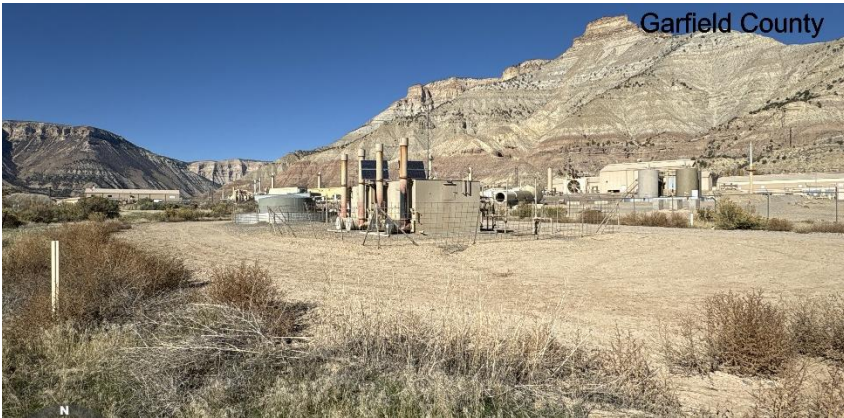
South West corner of location.
