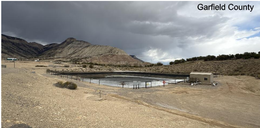
South West corner of location.
