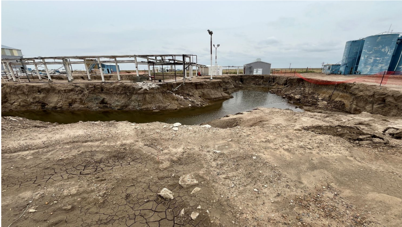
Photo 3. Facing north toward the remediation project.
