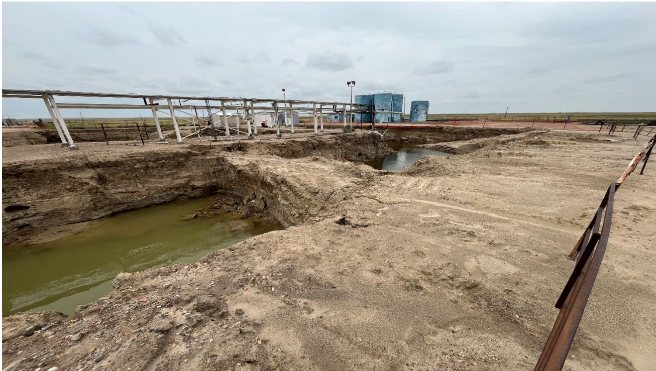
Photo 2. Facing northeast toward the remediation project.
