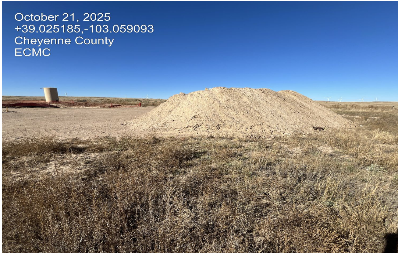
Photo 5. Facing north at the east side of the location. The fill material pile should have stormwater BMP's to prevent installed.
