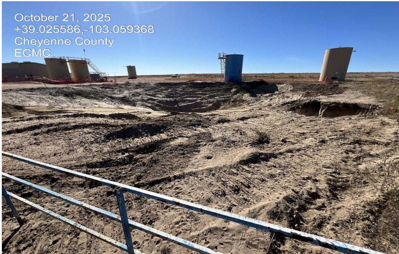
Photo 3. Facing west at the open excavation where tank battery was located.
