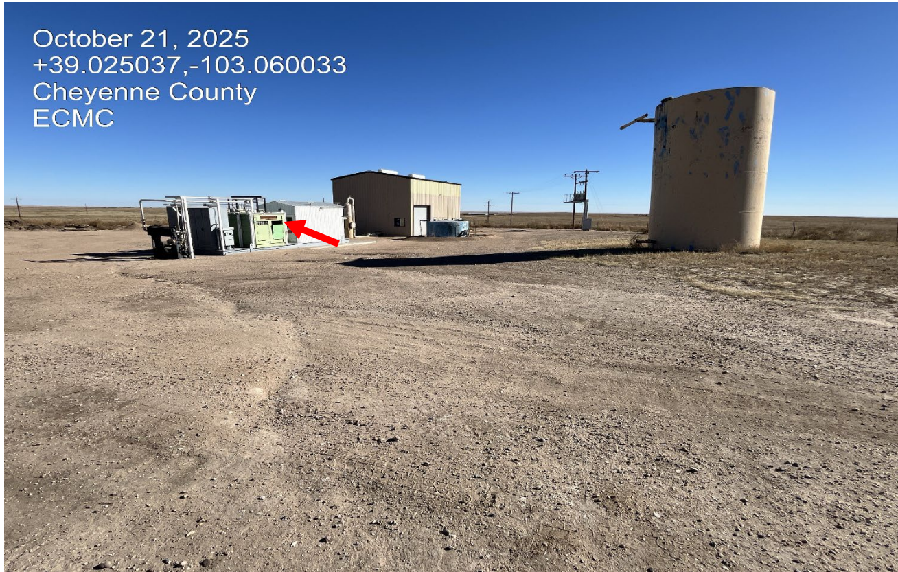
Photo 7. Facing southeast at the compressor facility.
