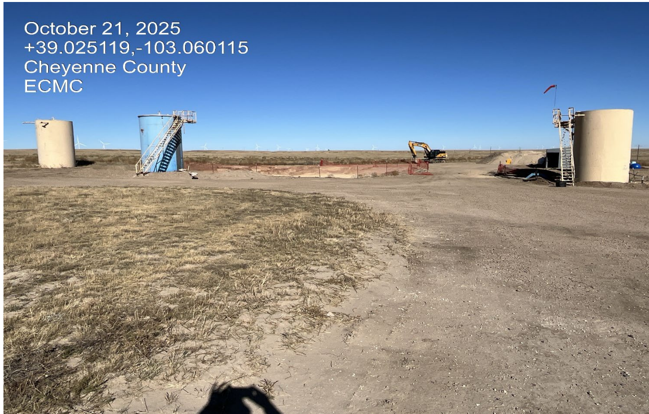
Photo 1. Facing northeast toward the tank battery facility.
