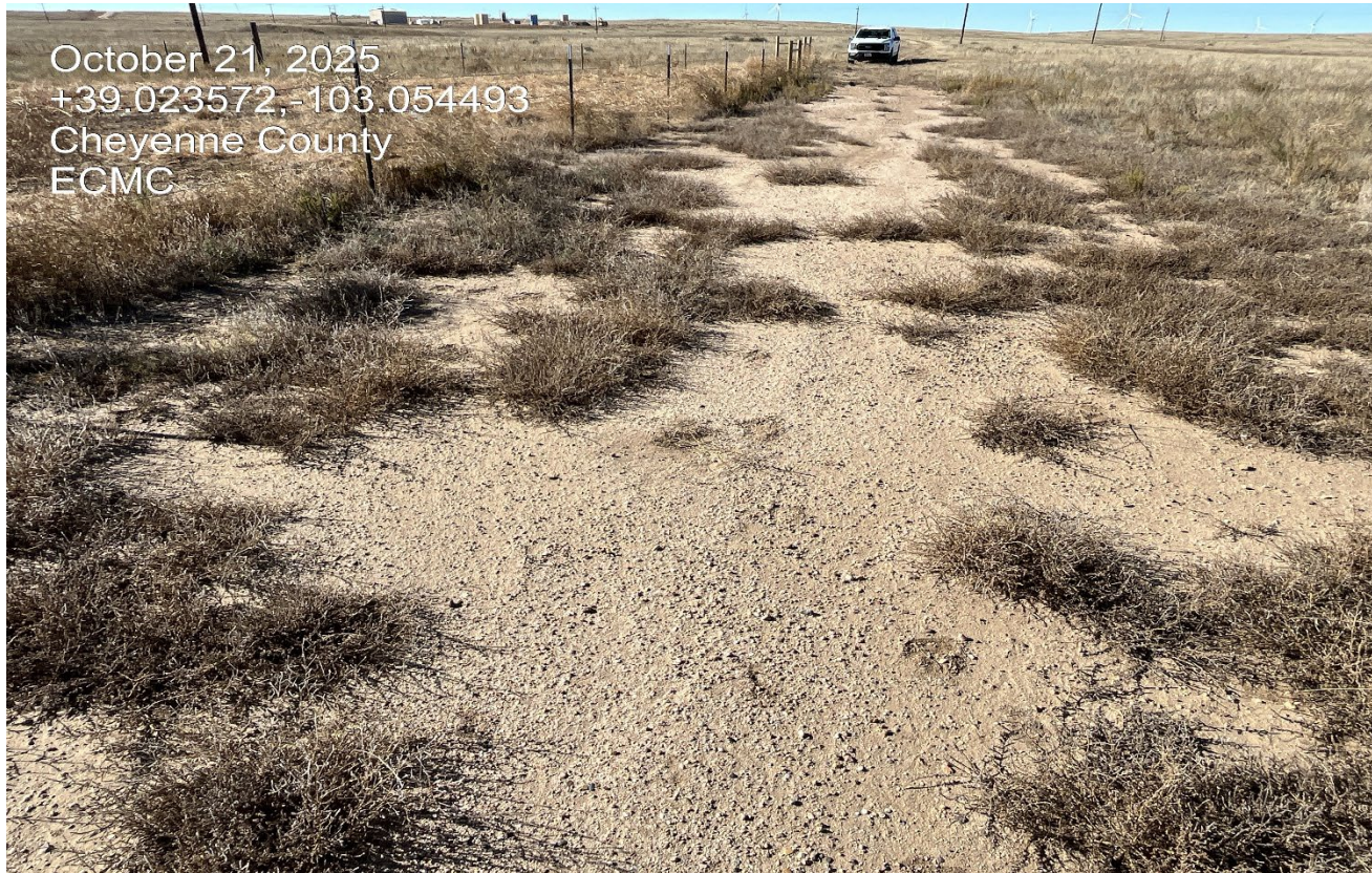
Photo 5. Facing north at the location. The access road continues thru the location however this area should be reclaimed back to a two track road.
