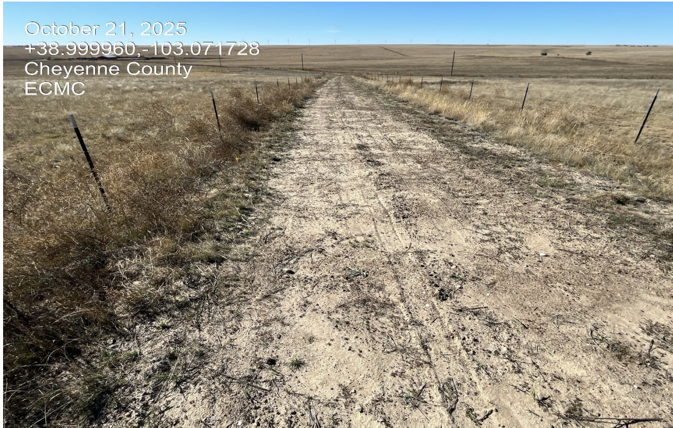
Photo 2. Facing west further along the road. The road was not regraded to match the surrounding contours and remains crowned with road side ditches.
