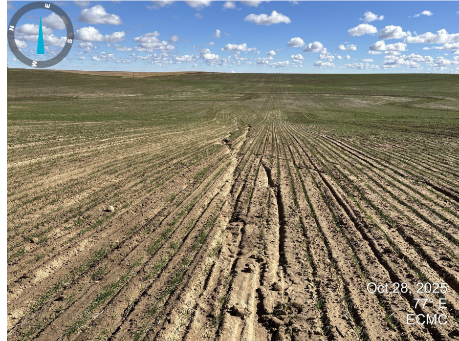
Photo 6. Looking east down the former access road towards the wellhead. Stormwater erosion is present along the former path of the access road.
