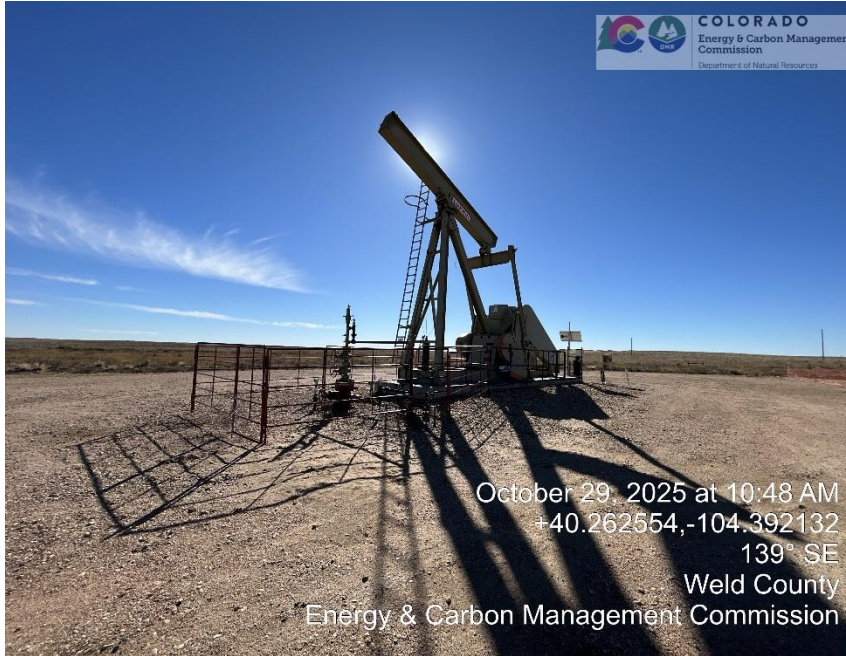
Unused pumping unit- no prime mover
