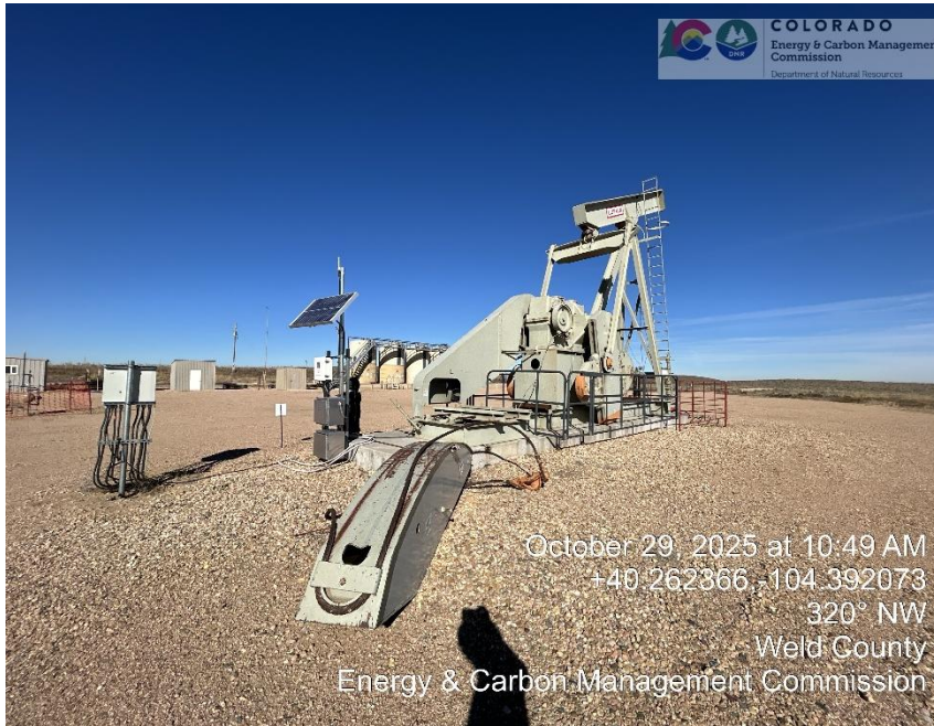
Unused pumping unit- no prime mover
